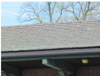
Ceramic tile roof in good condition
