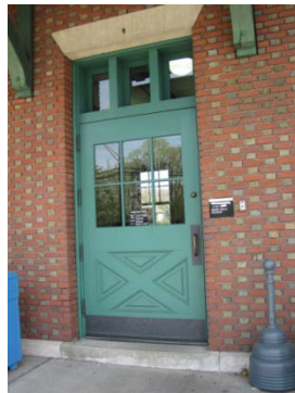
Exterior door good condition
