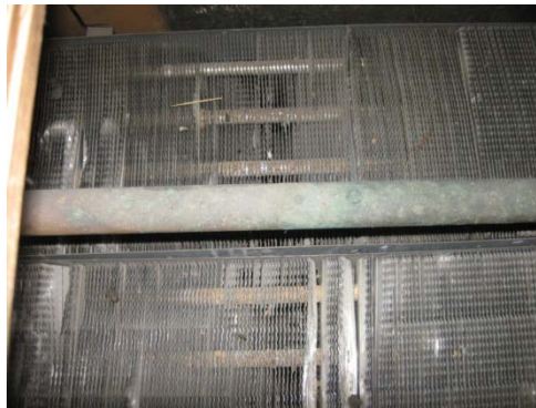
Radiators between waiting room benches
