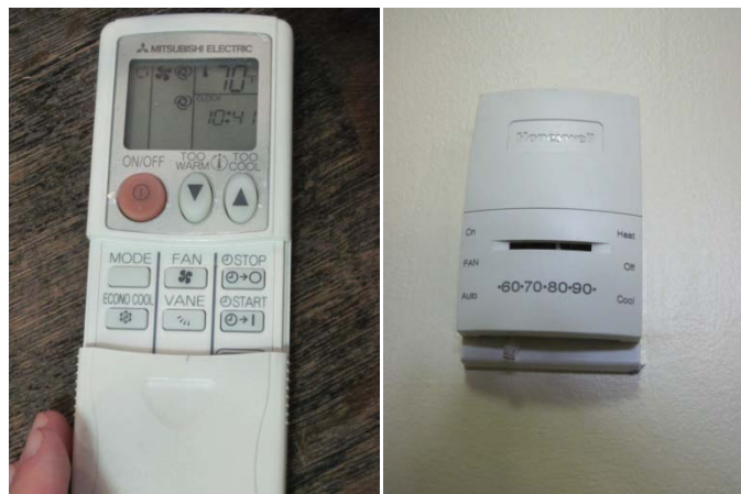
Hand held Mitsubishi thermostat for mini-split; Manual Honeywell thermostat for heating
