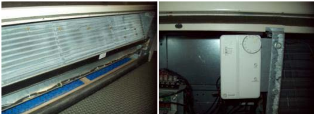
Inside of Trane unit ventilator (L); Thermostat on unit ventilator (R)
