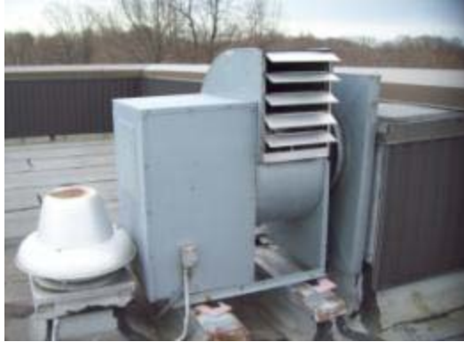
West wing roof-mounted corridor exhaust fan
