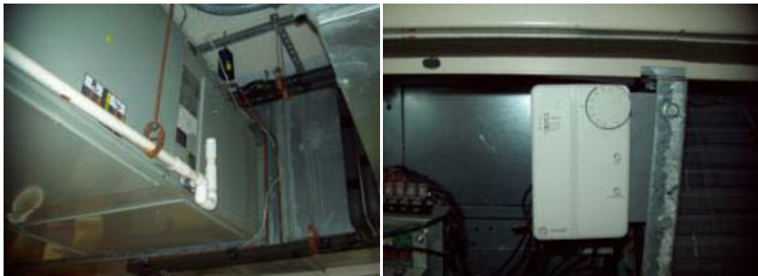
Trane air handling unit near Maintenance office (L); Connected Trane condenser (R)
