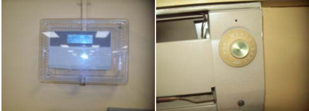
Common Area Programmable thermostat (L); Typical electric baseboard thermostat (R)
