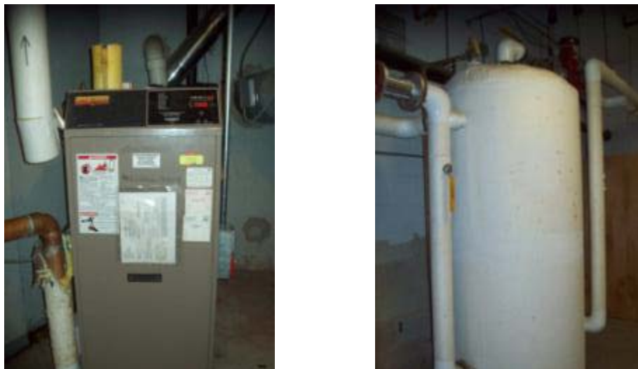
AO Smith – Burkay DHW heater (L); Approximate 400 gallon DHW storage tank (R)
