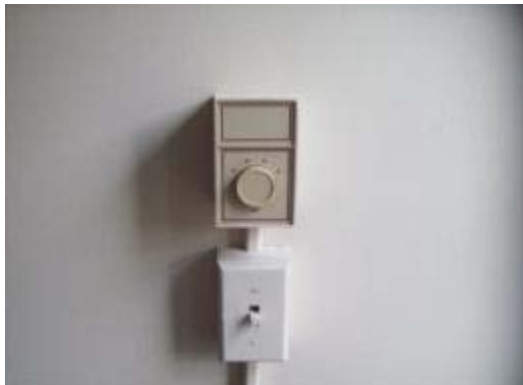
Non-programmable thermostat for electric baseboard heater
