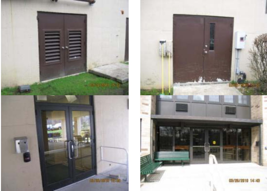
Missing/worn weather-stripping and damaged door frame
