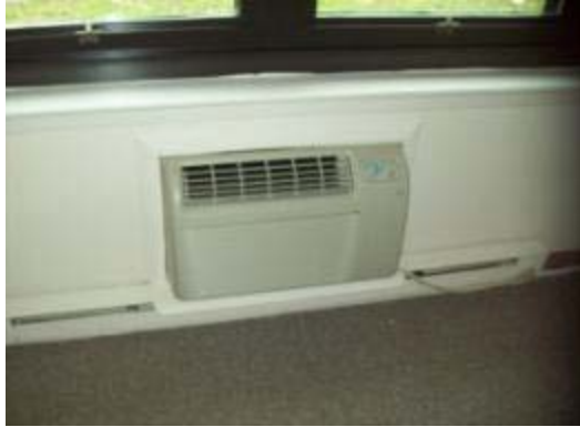
Electric baseboard and thru-wall AC unit in a typical apartment unit
