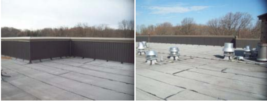
Typical roof surface with no signs of uncontrolled moisture, air-leakage or other energy-compromising issues
