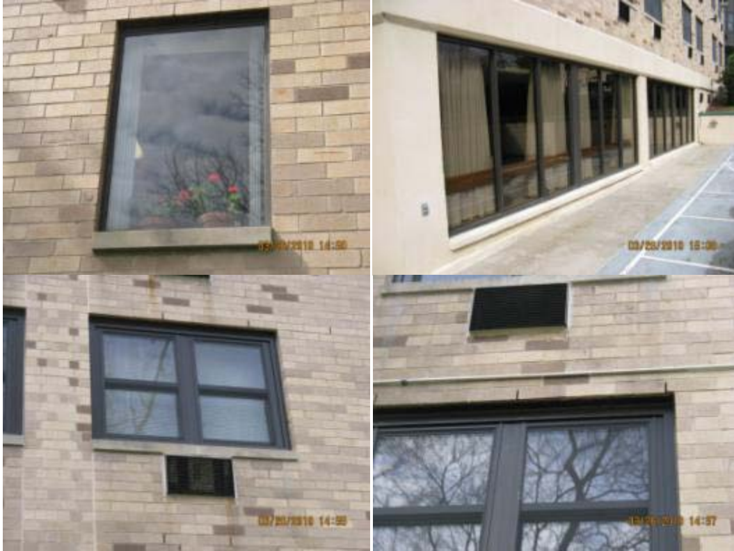
Cracked or aged caulk around frame/sill on the exterior
