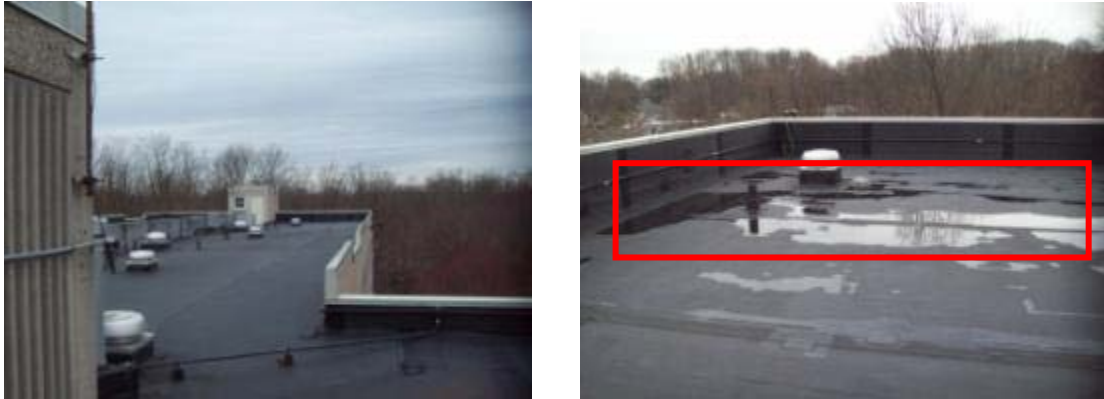
Signs of water pooling on the lower roof
