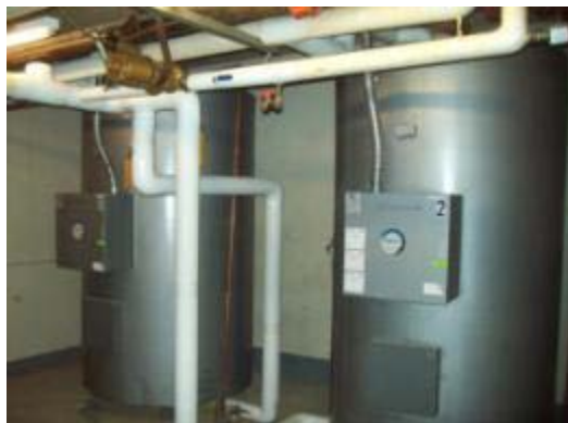
Two Hubbell electric DHW water heaters
