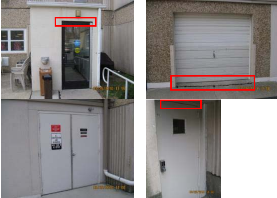
Missing/worn weather-stripping and damaged door frame.
