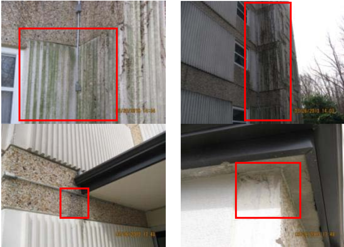
Signs of water damage, mold growth, overgrown vegetation, damage from roof runoff and damaged exterior wall surface.
