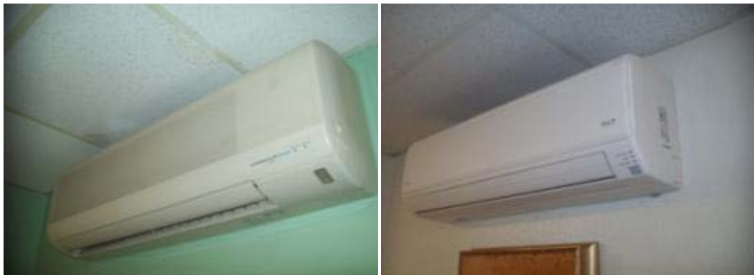
Evaporative Split AC units for Main Office (L); Community Room (R)
