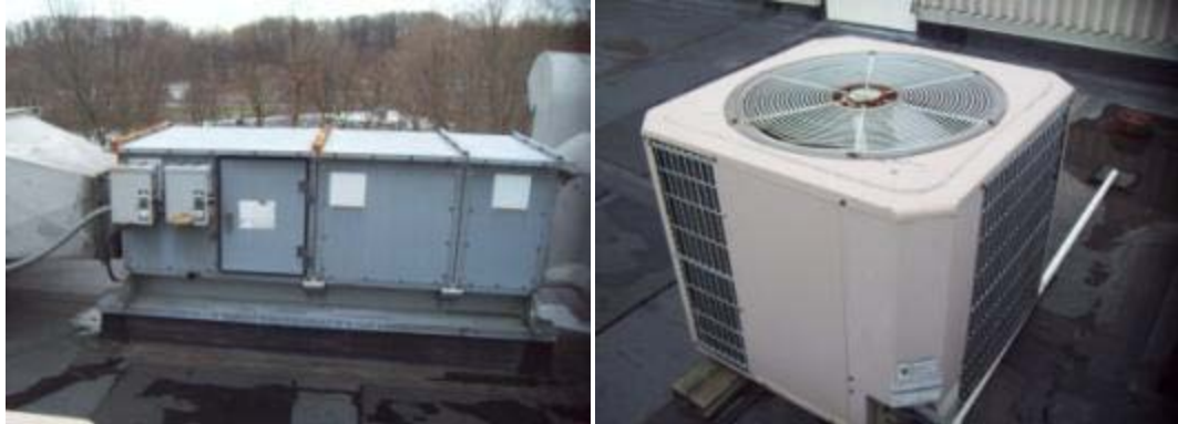
Trane rooftop unit (L); York condensing unit (R)
