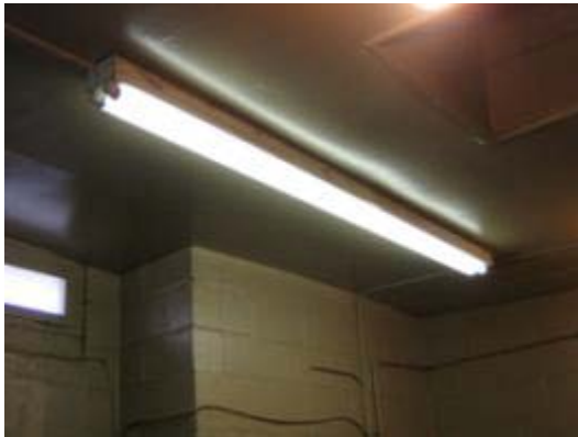
Surface-mounted fluorescent Light Fixture
