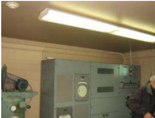
Surface-Mounted Fluorescent Light Fixture Above Pump Control Panel
