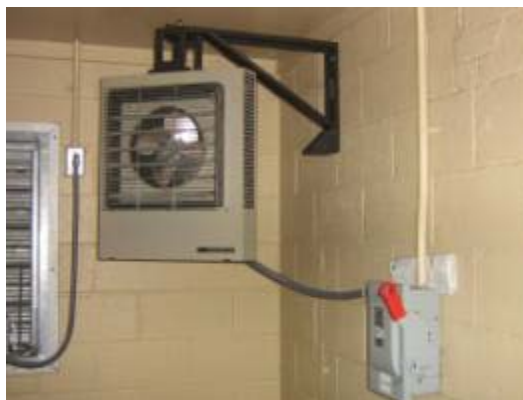
Electric Unit Heater
