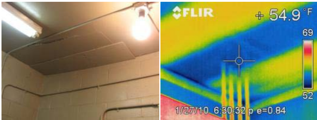
Digital Photo and Infrared Image of Plywood Panel
