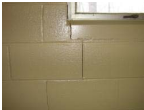
Through Wall Crack In Northwest Wall Of Deep Well
