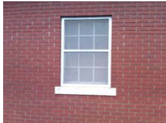
Typical windows and exposed window lintel that can lead to thermal bridging.
