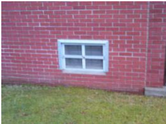
Typical windows and exposed window lintel that can lead to thermal bridging.
