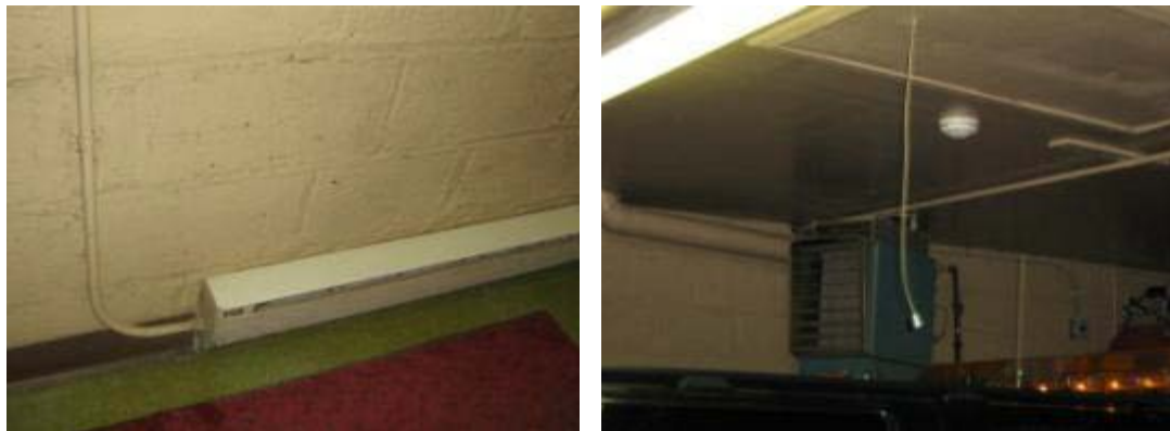
Electric baseboard heater, unit heater in garage
