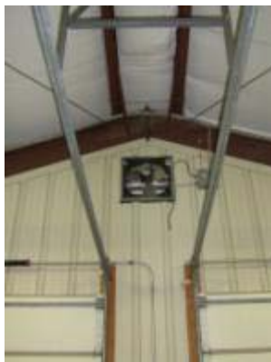
Exhaust fan in peak of structure, motorized louver in rear of space
