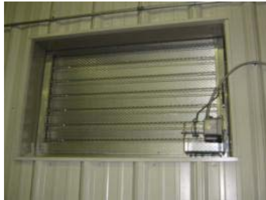
Exhaust fan in peak of structure, motorized louver in rear of space
