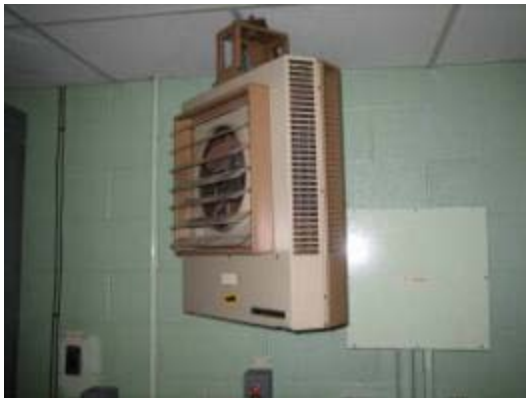
Electric unit heater in Effluent Pump Station
