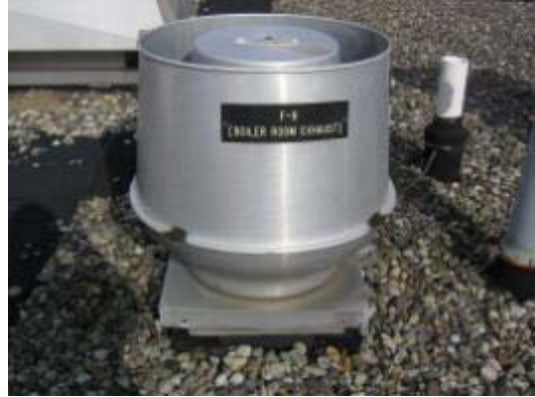
Various exhaust fans and HV-3 unit; Close-up of F-9 boiler room exhaust fan
