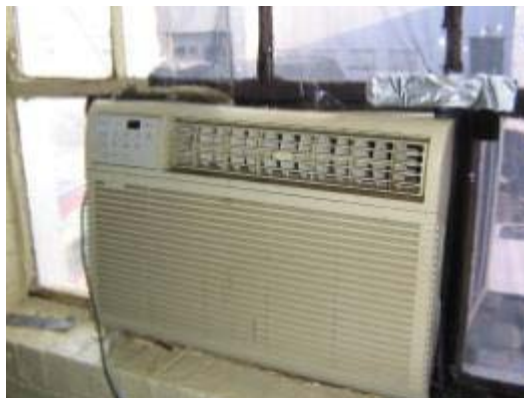
Thru-wall AC unit
