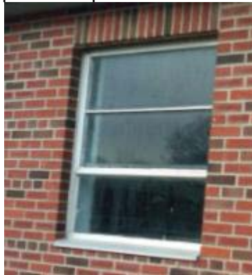
Typical window installation with exposed lintel
