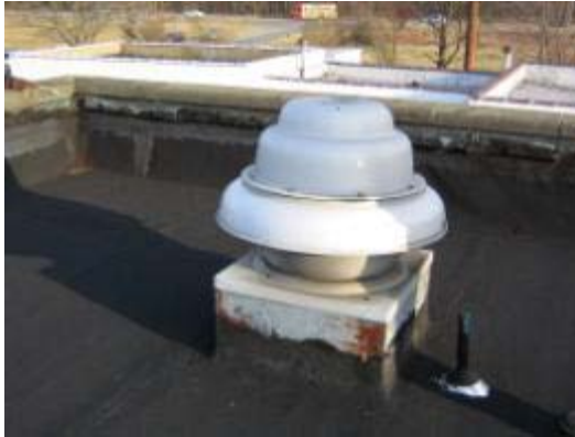
Roof mounted exhaust fan
