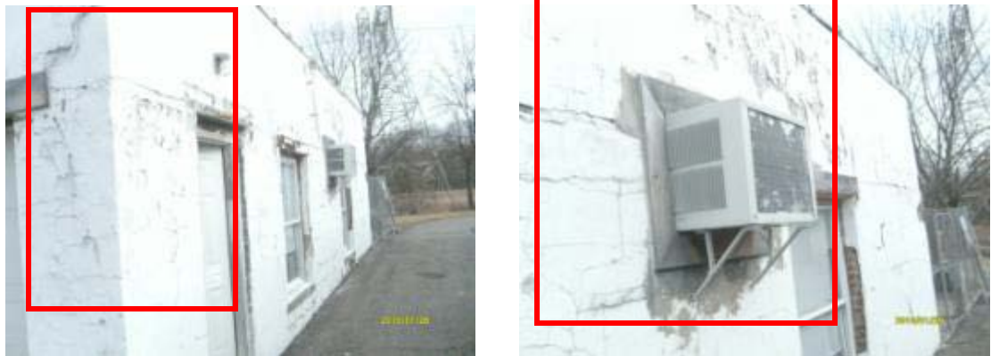
Damaged exterior wall finishes, uncontrolled roof water run-off due to defective/ clogged gutters and downspouts and un-caulked/ un-sealed exterior wall penetrations
