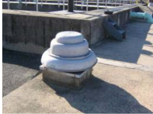
Roof of Maintenance building; Exhaust fan for underground tunnel
