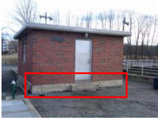
Typical exterior wall finish and signs of water damage at building grade
