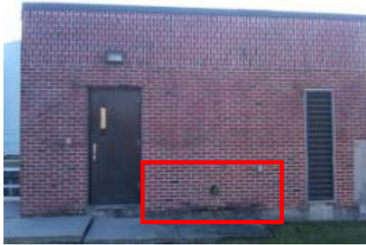
Cracked/ deteriorated bricks and mortar joints, exposed building penetration, and signs of water damage at perimeter walls due to missing/ ineffective site drainage
