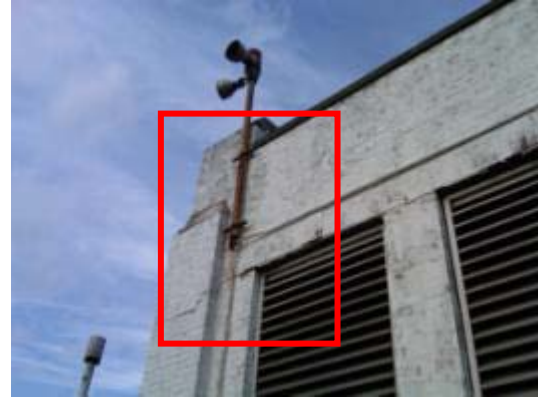
Identified areas of shifted brick, water damage and cracked caulking.
