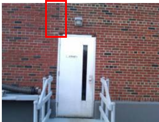
Maintenance building with cracked and missing caulking, and damaged exterior wall finish
