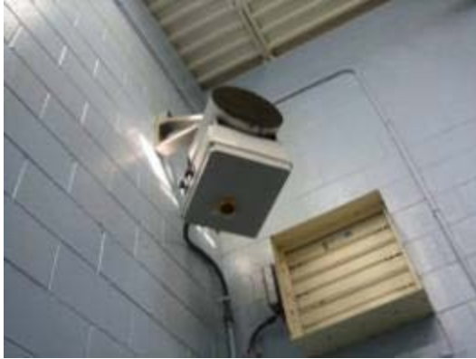
Electric unit heater
