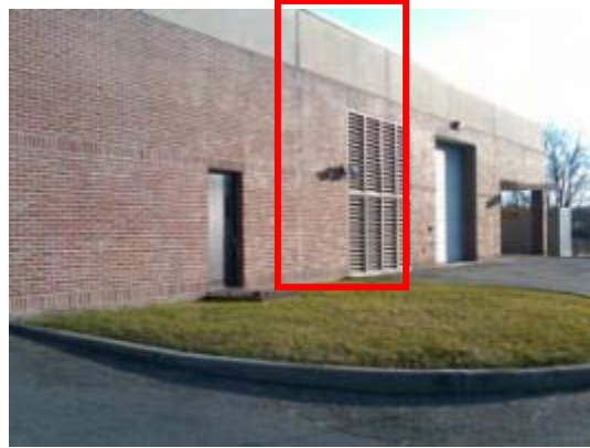
Signs of water damage at perimeter walls due to missing/ ineffective site drainage and cracked/ aged caulk
