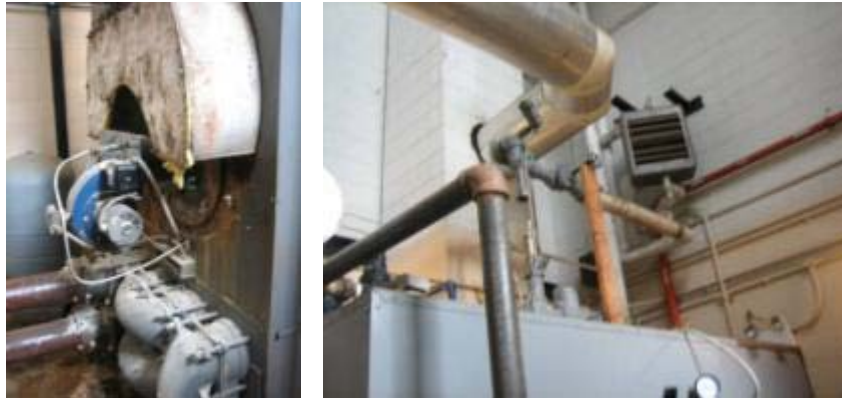
Hot water boiler; Hydronic unit heater
