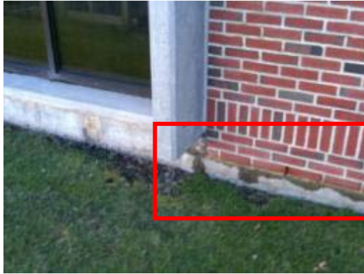
Signs of water damage at perimeter walls due to missing/ ineffective site drainage and cracked/ aged caulk
