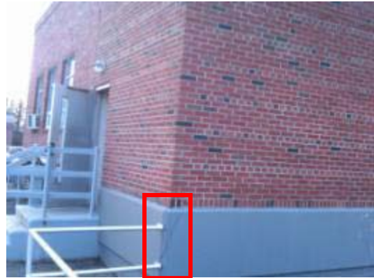
Maintenance building with cracked and missing caulking, and damaged exterior wall finish
