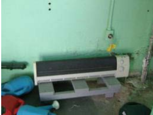
Portable electric baseboard heater
