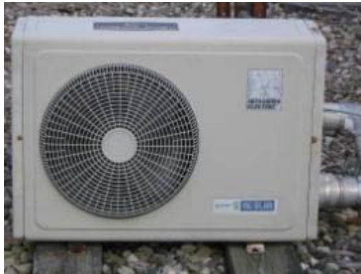
Air-cooled condensing unit on roof for Control Room cooling
