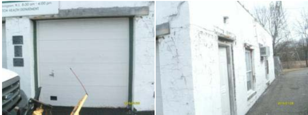
Typical exterior doors with damaged frames
