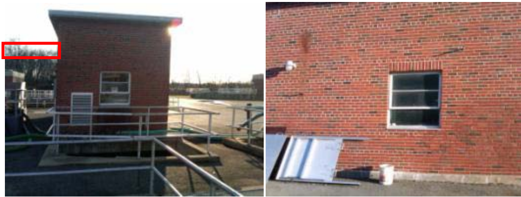
Damaged/aged window frame exposed window lintel, missing window sill and drip-edge detail
