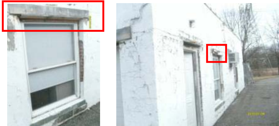
Typical window installation and signs of damaged window frames, infiltration and water damage.
