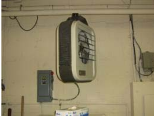
Electric unit heater
