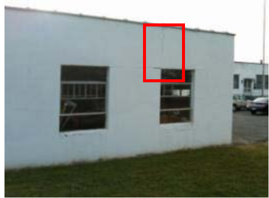
Damaged exterior wall finish
