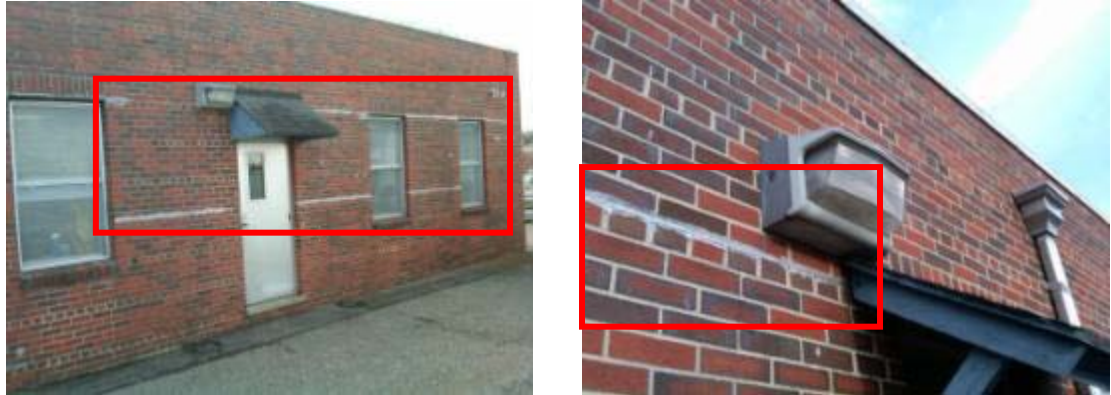
Identified areas of efflorescence crack caulking.
