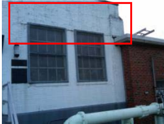
Identified areas of shifted brick, water damage and cracked caulking.
