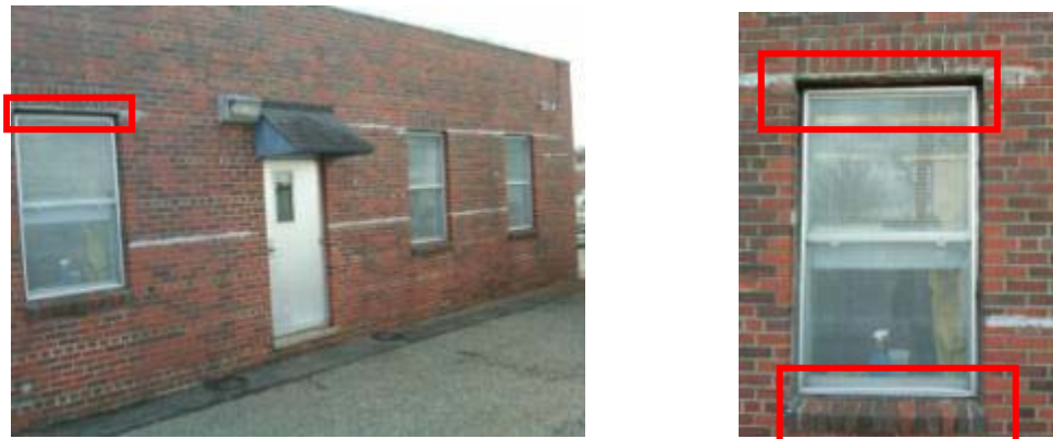
Damaged/old window frame exposed window lintel, missing window sill and drip-edge detail
