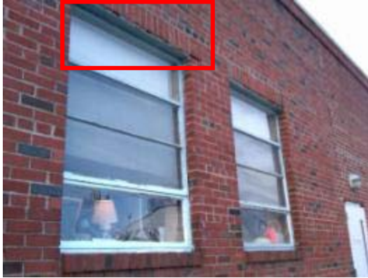
Typical window with exposed window lintel,
