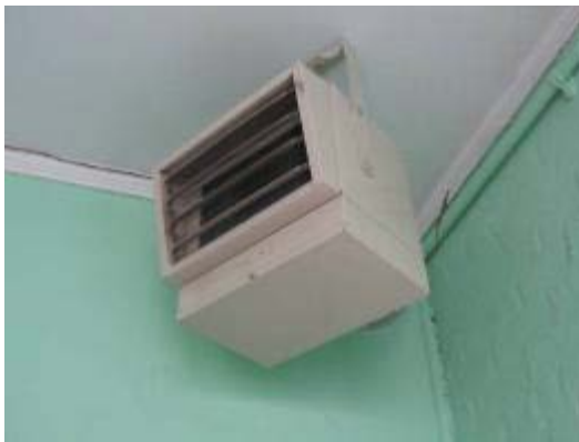
Electric unit heater in locker room
