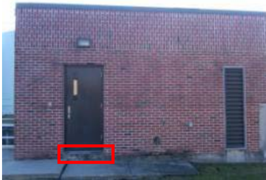
Typical exterior door with damaged lower portion of door frame
