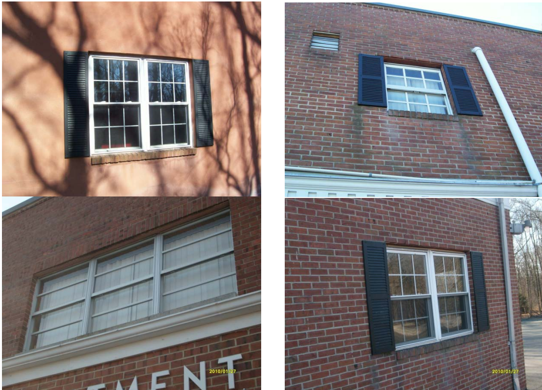
Windows with exposed lintels and signs of water damage at sills and storm doors
