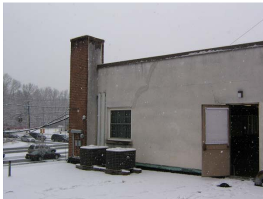
Split system condensing units on roof
