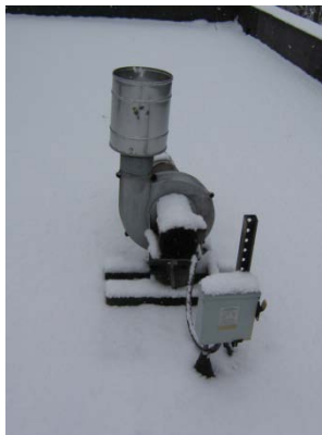
Vehicle exhaust fan on roof
