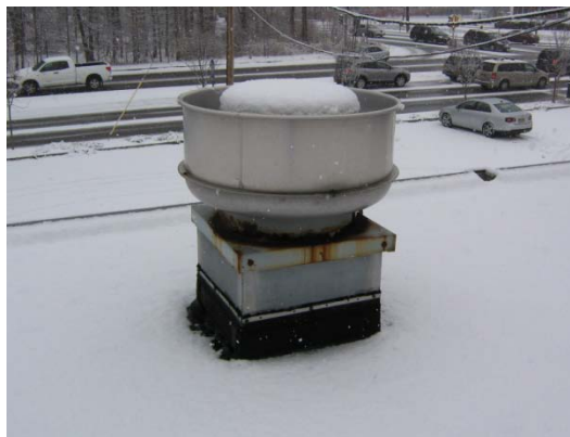
Kitchen hood exhaust fan on roof
