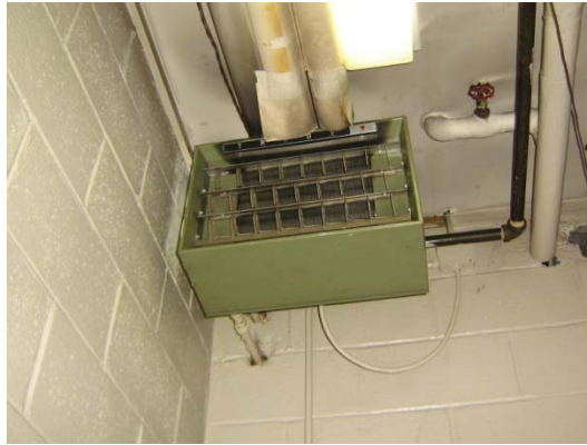
Typical unit heater in Garage.
