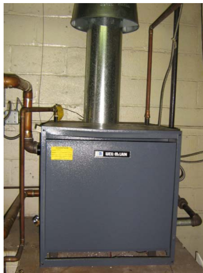
Gas fired boiler in Boiler Room
