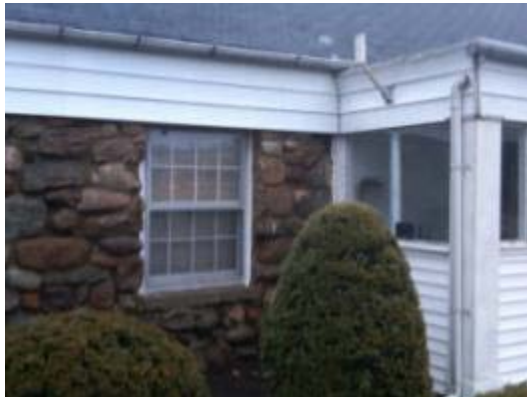
Partial West Façade
