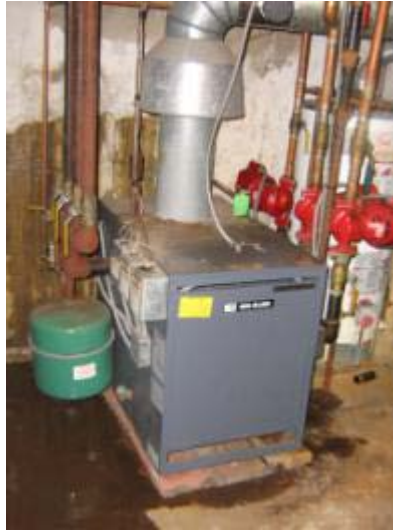
Gas fired boiler and three heating hot water supply pumps in basement
