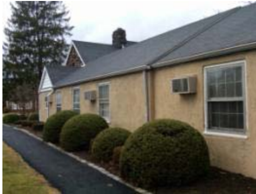
Partial South Façade
