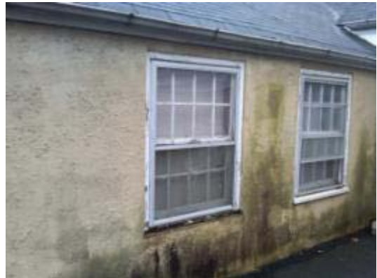
Partial North Façade
