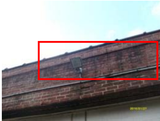
Examples of water damage, displaced masonry units and cracked caulking
