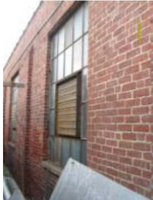
Typical window installations and examples of damaged frames sills and cracked glazing.
