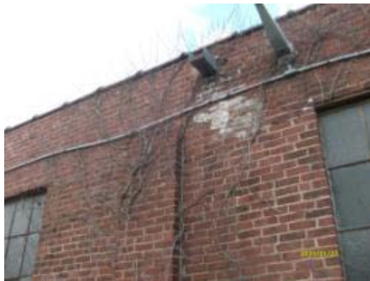
Efflorescence on brick and masonry walls indicate moisture presence within the wall cavity. and signs of plant overgrowth
