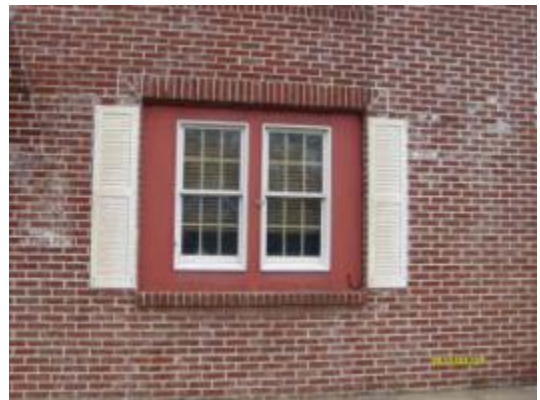
Efflorescence on brick and masonry walls indicate moisture presence within the wall cavity. and signs of plant overgrowth
