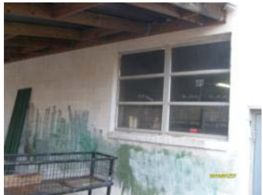
Partial North Façade
