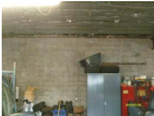
Typical Unfinished interior concrete block wall
