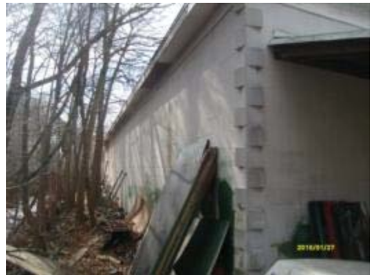
Partial East Façade
