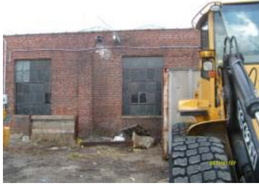
Partial South Façade
