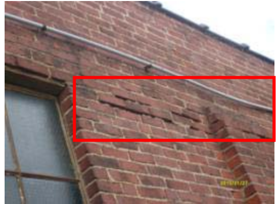
Examples of water damage, displaced masonry units and cracked caulking
