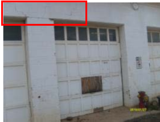
Cracked/ aged caulk, cracked concrete blocks and signs of water damage from roof drainwater run-off.due to defective flashing and gutters.
