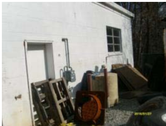
Partial South Façade
