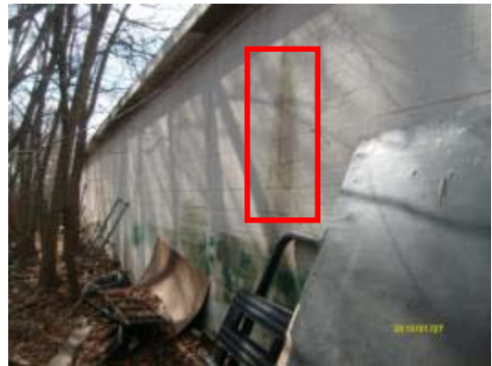
Cracked/ aged caulk, cracked concrete blocks and signs of water damage from roof drainwater run-off.due to defective flashing and gutters.
