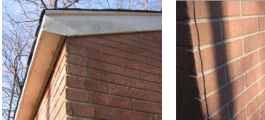
Severe Cracks Through Veneer (Left); Typical Vertical Crack (Right)
