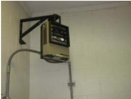
Electric Unit Heater in Pump Control Room
