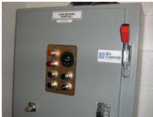
Controls for One of the Sewage Pumps
