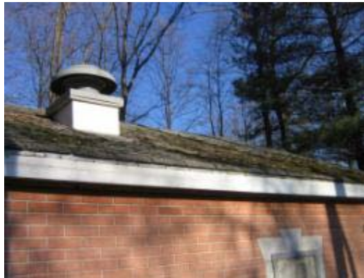
Deteriorated Roof Shingles
