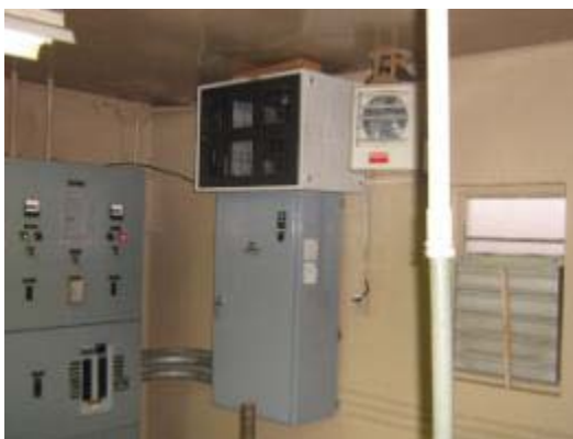
Electric Unit Heater to Left of Vertical Pipe and Window Louver to Right
