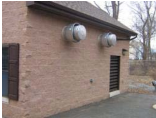
Wall-Mounted Exhaust Fans
