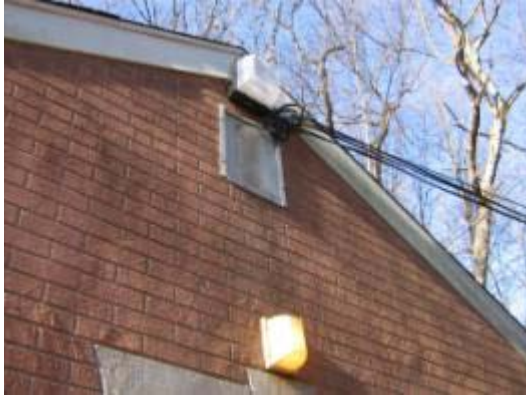
Metal Halide and Incandescent Fixtures Above Front Door
