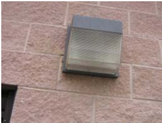
Exterior Metal Halide Wallpack Light Fixture
