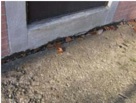
Cracked base at south wall
