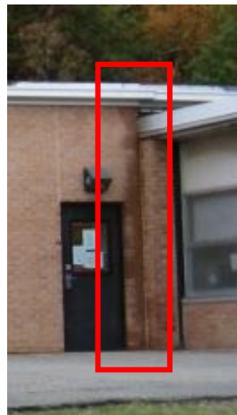
Water infiltrated veneer caused by faulty flashing
