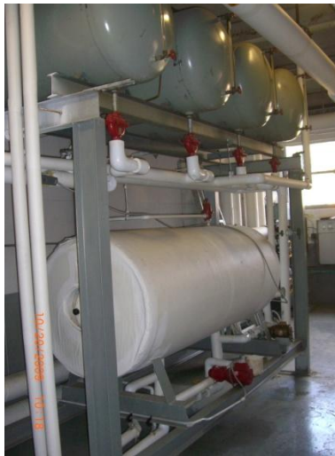
Domestic Water Storage Tank with Expansion Tanks Above
