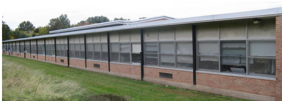
Older aluminum window wall section
