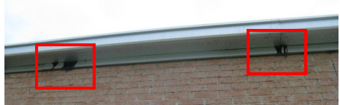
Roof tar melting on exterior and interior of building
