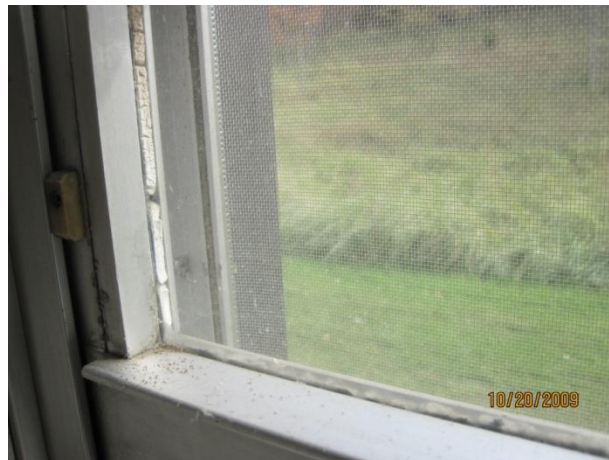
Older windows showing cracked and damaged caulk
