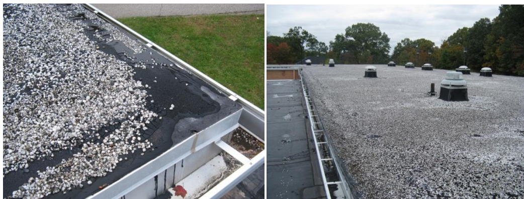
Built up roof area showing tar run-off into and behind gutters
