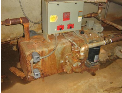
Duplex Condensate Receiver Pump Set In Boiler Room
