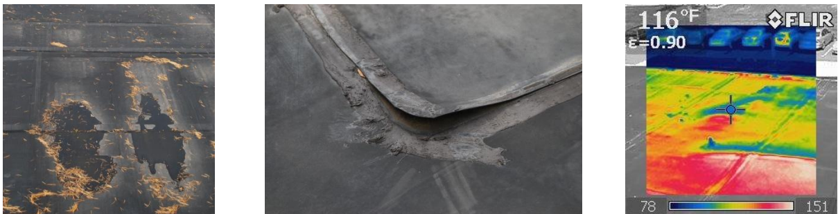
Signs of pooling, cracked EPDM seams and dry cold spots
