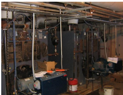
Two of the Three Steam Boilers
