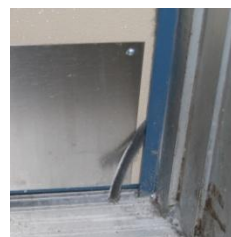
Signs of worn or missing weather stripping
