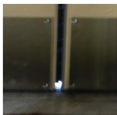
Signs of worn or missing weather stripping
