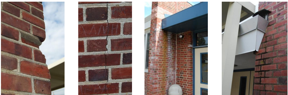
Cracked caulk, bricks and mortar together with signs of uncontrolled roof water were found
