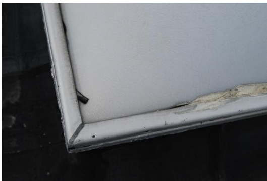
Skylight and window caulking showing signs of age
