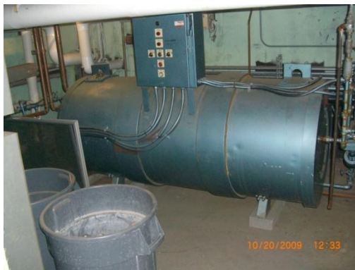
Boiler Feed-water Tank
