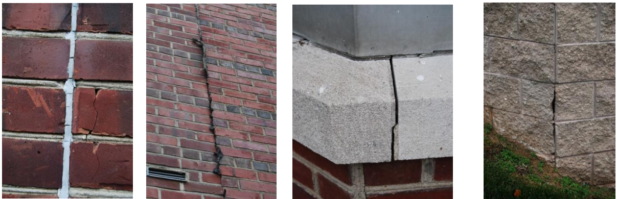
Cracked caulk and mortar, inappropriate filler materials were found in isolated areas
