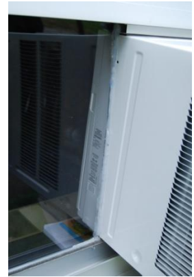
Windows showing damaged glass and air conditioning units with inefficient seal
