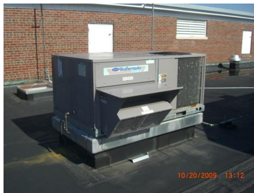
Packaged HVAC Rooftop Unit Serving Front Offices, Nurse's Office and SGI
