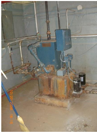
Duplex Condensate Receiver Pump Set In Boiler Room
