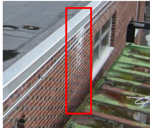
Stairwell wall showing crack Un-controlled roof water runoff caused by cap flashing failure
