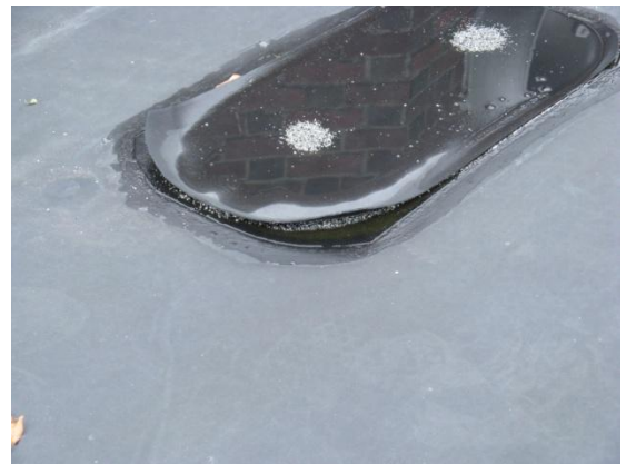
1990 EPDM roof showing pooling post rainfall; Un-sealed seam on same roof area
