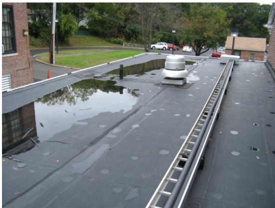
1990 EPDM roof showing pooling post rainfall; Un-sealed seam on same roof area
