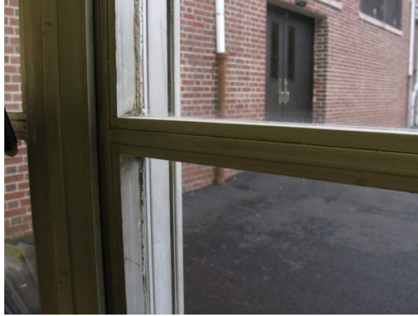
Older windows showing cracked and damaged seals
