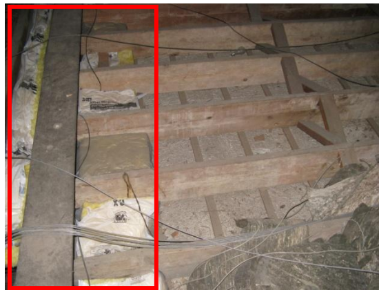
1" faced batt insulation and attic bays without insulation in 1929 section of building
