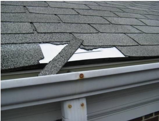
Asphalt roof section showing damaged shingle
