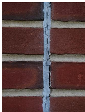
Cracked caulk, inappropriate filler materials and surface algae growth due to uncontrolled roof water run off
