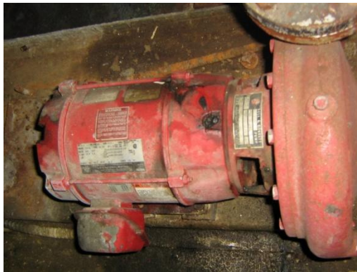
Hot Water System Circulating Pump
