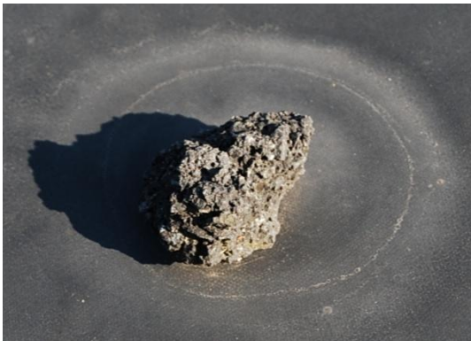
Sharp edge rocks and vegetation can impact roof finish warranties and life-span
