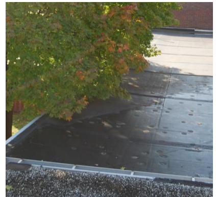
Sharp edge rocks and vegetation can impact roof finish warranties and life-span
