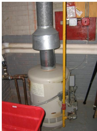
Photo – Burkey type domestic water heater
