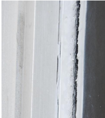
Window caulk showing cracks
