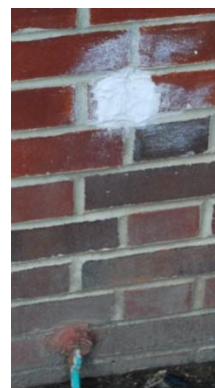
Cracked caulk, inappropriate filler materials and surface algae growth due to uncontrolled roof water run off
