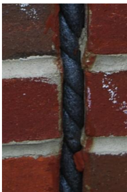
Cracked caulk, inappropriate filler materials and surface algae growth due to uncontrolled roof water run off
