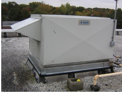
Heating Only RTU serving 2002 Gym Addition
