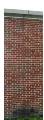
Cracked caulk, inappropriate filler materials and surface algae growth due to uncontrolled roof water run off
