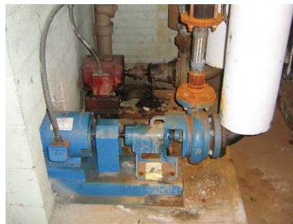
Corrosion evident on pump bodies and piping connections
