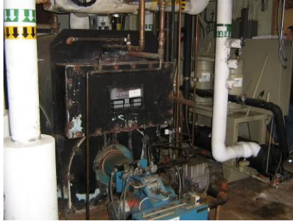
Original 1968 firebox boiler
