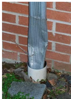
Damaged and disconnected downspouts
