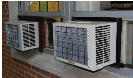
Window air conditioning units sealed with thermal tape
