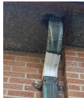
Damaged and disconnected downspouts
