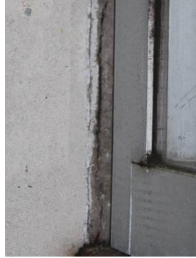
Window caulk showing cracks
