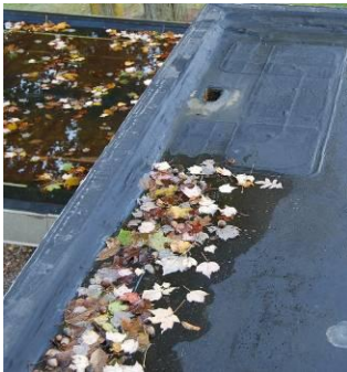
Pooling and IR images showing signs of no or little roof insulation
