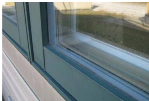
(Photo showing new thermo pane windows.)
