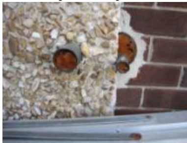
Annular space between pipes is not sealed
