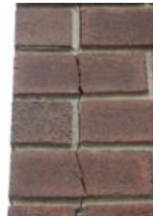
Cracked Brick
