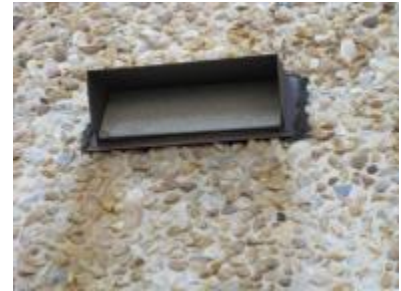
Failed Perimeter Sealant
