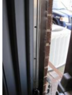
Worn Weather-stripping
