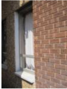
Cracked Sealant
