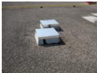
Abandoned Exhaust Fans Not Insulated
