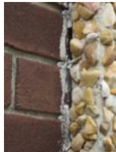
Failed Perimeter Sealant
