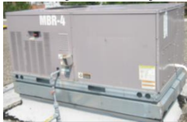
Carrier packaged rooftop DX unit
