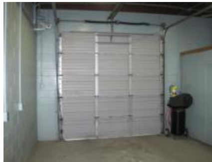
Un-insulated, No Weather-stripping
