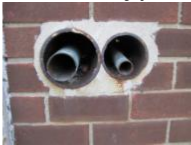
Annular space between pipes is not sealed
