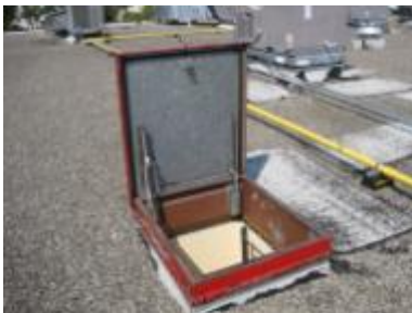
Roof Hatch Not Insulated
