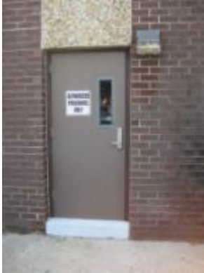
No Threshold or Weather-stripping
