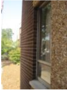
Cracked Sealant
