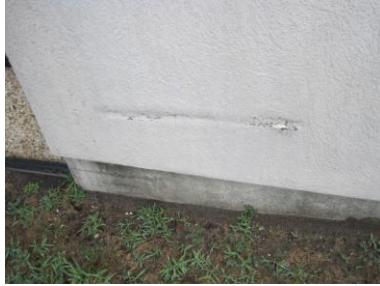
Damaged EIFS System
