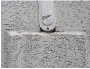
Gaps in sealant at penetrations
