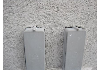
Gaps in sealant at penetrations
