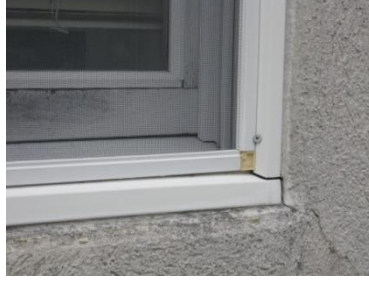
Deteriorated sill and window. Frame components need sealant Air leakage is occurring at sill. Hermetic seal broken at lower sash.
