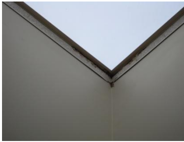
Rust stains indicating condensation due to single glazed skylight
