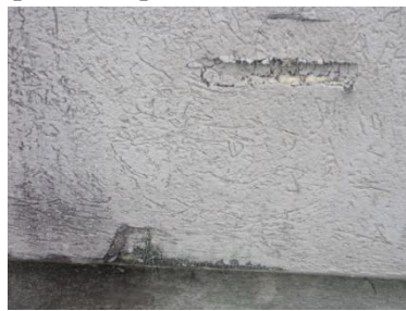
Damaged EIFS System
