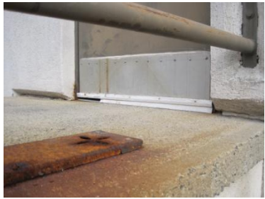
Missing weather-stripping
