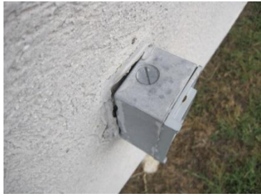
Gaps in sealant at penetrations
