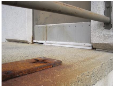
Missing weather-stripping
