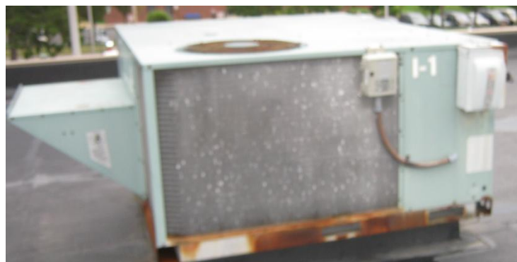
Carrier packaged rooftop DX unit
