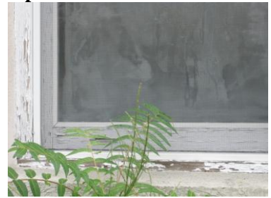
Deteriorated sill and window
