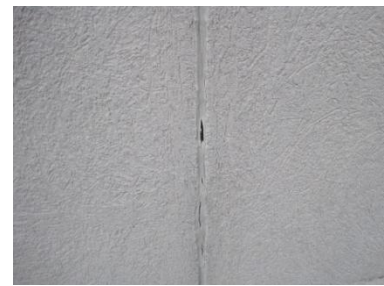
Gaps in sealant at panel joints
