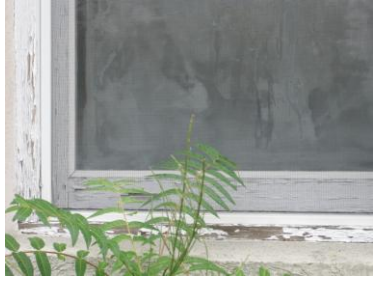
Deteriorated sill and window. Frame components need sealant Air leakage is occurring at sill. Hermetic seal broken at lower sash.
