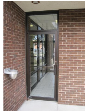
Missing weather-stripping at door bottom, integral door weather-stripping is worn
