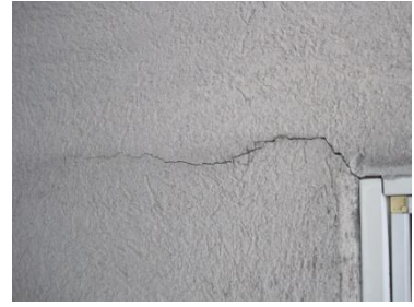
Frame to EIFS joints need to be sealed
