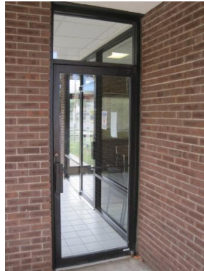
Missing weather-stripping at door bottom, integral door weather-stripping is worn
