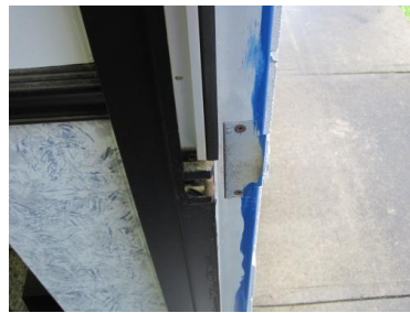
No Weather-stripping on Bottom Half of Jamb
