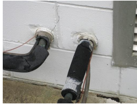
Bldg. Crack & Aged Sealant
