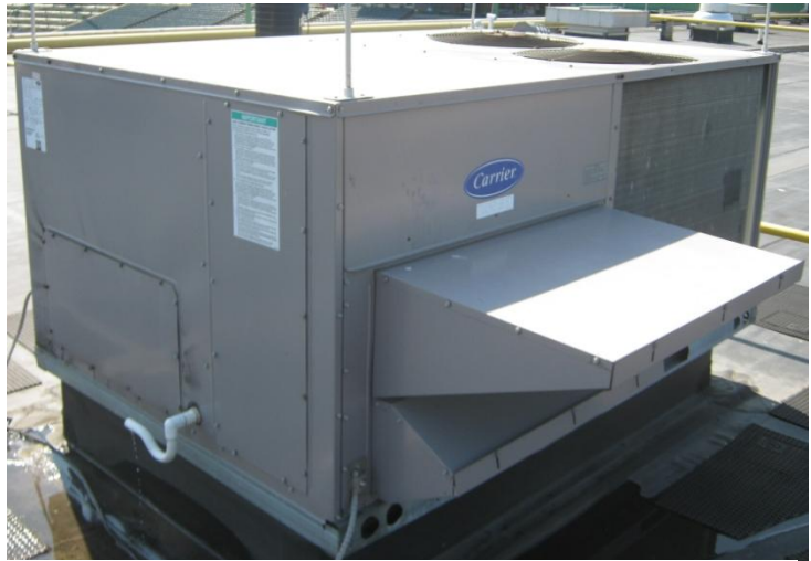
Carrier packaged rooftop DX unit
