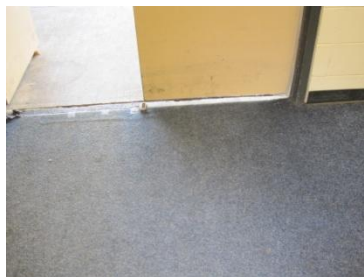
No Threshold/No Weather-stripping
