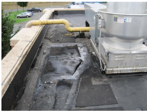
Membrane Deterioration over Kitchen Due to Grease Exhaust
