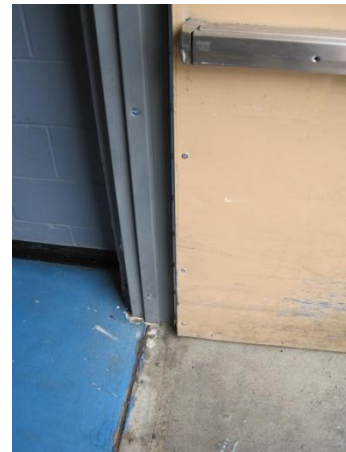
No Threshold/No Weather-stripping
