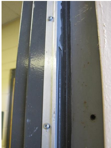
Worn Weather-stripping
