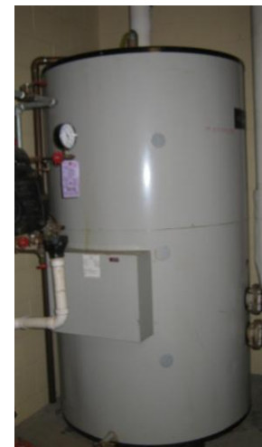
Lochinvar 400-gallon domestic hot water tank
