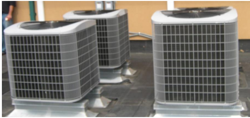
Carrier split-system heat pumps
