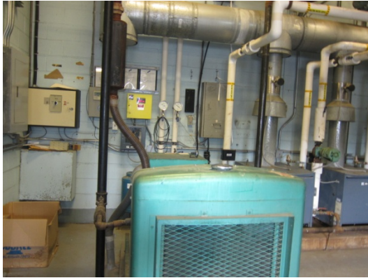
25 kW natural gas generator
