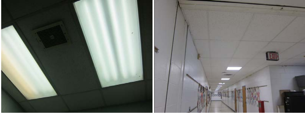
Typical interior linear and u-shaped T8 fixtures
