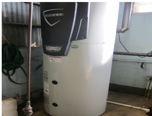
Lochinvar Condensing DHW heater
