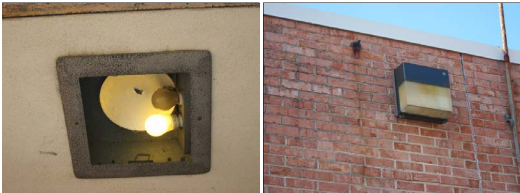
Typical recessed CFL and high pressure sodium wall pack fixtures. Note: The fixture on the left is operating during daytime hours due to incorrect time clocks
