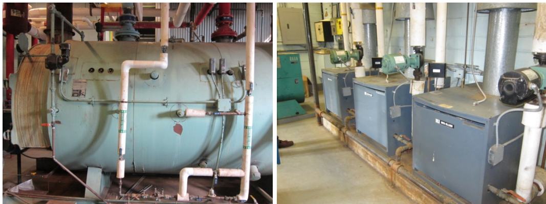
American Standard - Kewanee boiler – old section (L); 3 Weil-McLain boilers – new section (R)
