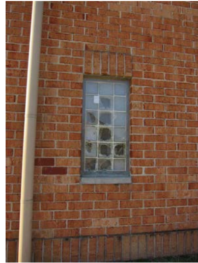
Typical single-hung type window with a non-insulated frame(L) and broken glass block windows in gymnasium(R)
