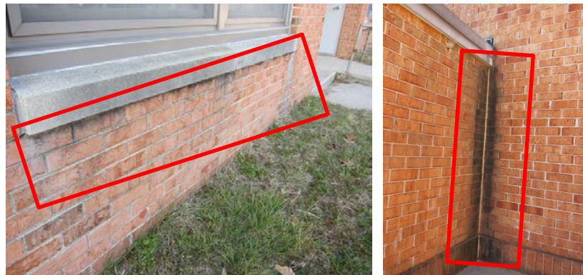
Efflorescence beneath window sill indicates moisture in the wall and uncontrolled roof run-off due to defective/clogged gutters and downspouts
