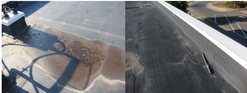
Pooling/standing water and roof debris
