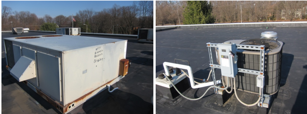
Typical rooftop unit (L); View of typical rooftop condensers for unit ventilators (R)
