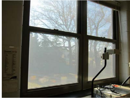
Typical single-hung type window with a non-insulated frame(L) and broken glass block windows in gymnasium(R)
