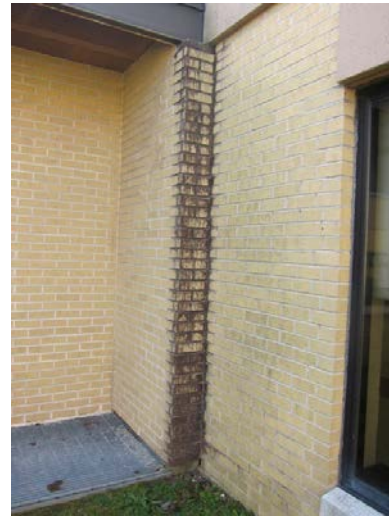
Deteriorating bricks, unsealed wall penetrations and signs of uncontrolled roof water runoff
