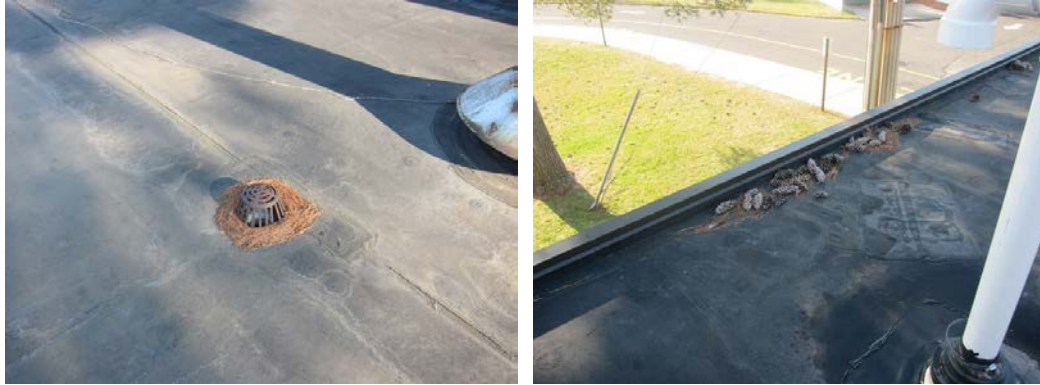
Pooling/standing water and foliage clogging roof drains
