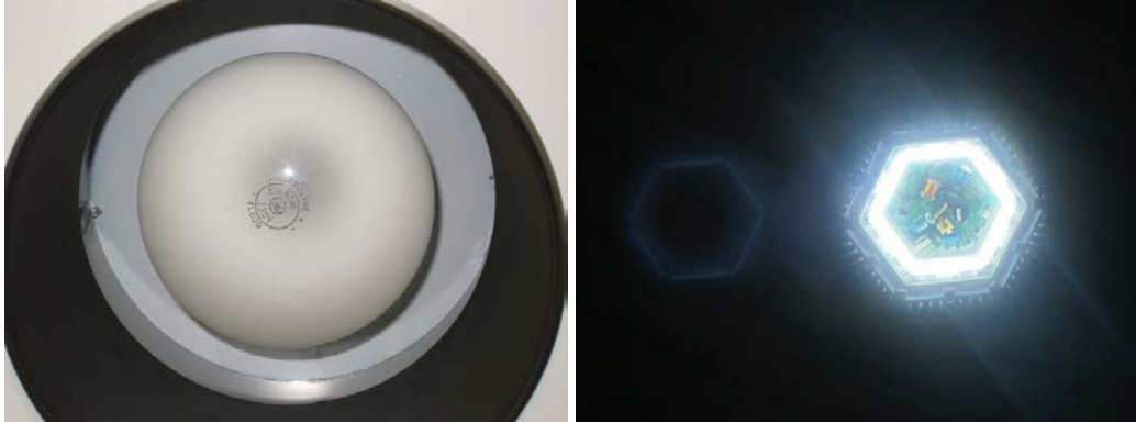
Incandescent flood lamps found in the library and LED fixtures found in the gymnasium
