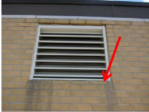
Efflorescence on brick and masonry indicate moisture presence within the wall cavity
