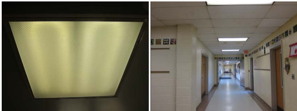
Typical interior u-shaped and linear T8 lighting
