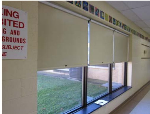
Typical fixed type windows with a non-insulated frame
