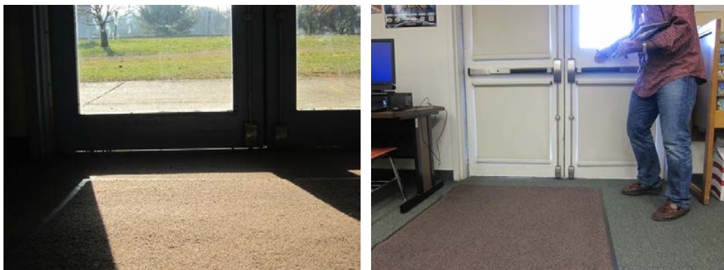
Missing/worn weather-stripping
