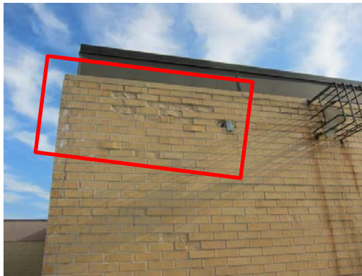
Deteriorating bricks, unsealed wall penetrations and signs of uncontrolled roof water runoff
