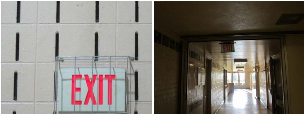
Typical new LED exit sign (L) and typical old LED exit signs (R)
