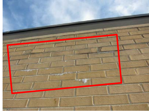
Efflorescence on brick and masonry indicate moisture presence within the wall cavity
