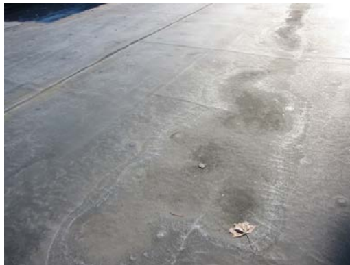
Signs of pooling/standing water were found throughout all the roof surfaces
