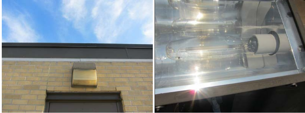
Typical high pressure sodium wall pack and spotlight fixtures
