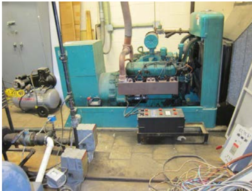
85 kW natural gas generator
