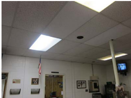
Typical interior T8 lighting)
