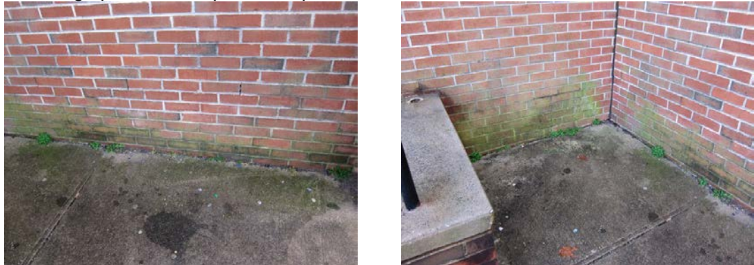
Biological growth due to poor sight drainage
