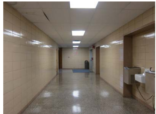
Typical interior T8 lighting in classrooms and hallways
