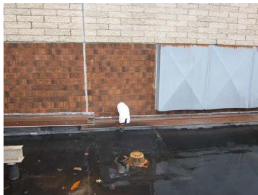
Pooling/standing water at the base of the Westinghouse dry cooler (L), and foliage on roof surface may lead to clogged roof drains (R).
