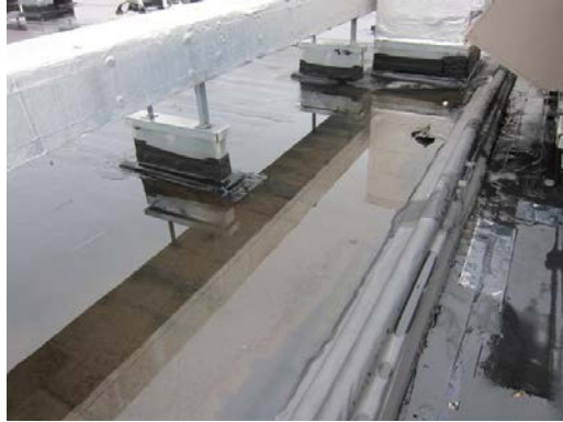
Pooling/standing water (L), and foliage on roof surface has clogged roof drains (R).
