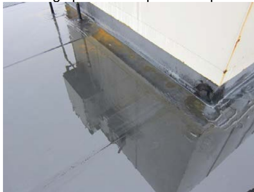
Pooling/standing water at the base of a roof top unit (L), and foliage on roof surface may clog roof drains (R).
