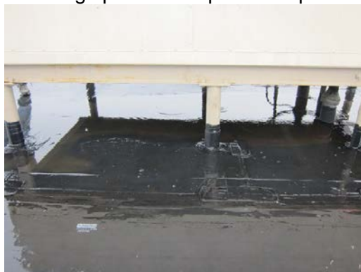
Pooling/standing water at the base of the Westinghouse dry cooler (L), and foliage on roof surface may lead to clogged roof drains (R).
