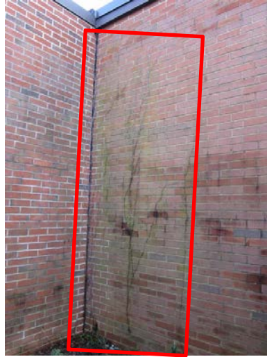
Overgrown ground vegetation touching exterior wall surfaces indicates moisture in the wall and contributes to façade deterioration
