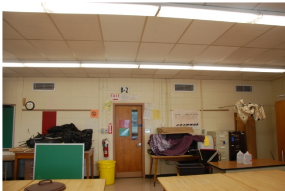
Typical interior T8 lighting in classrooms and hallways
