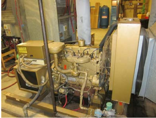
30 kW natural gas generator
