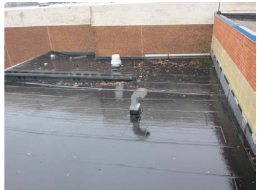
Pooling/standing water at the base of a roof top unit (L), and foliage on roof surface may clog roof drains (R).
