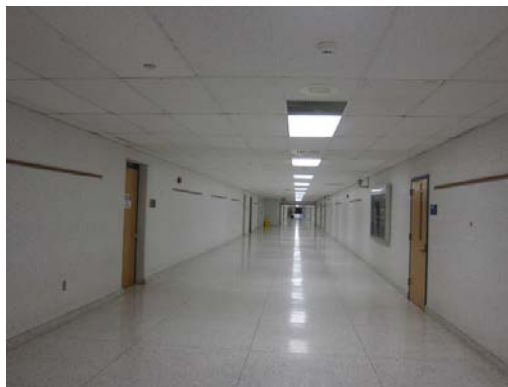
Typical interior T8 lighting)
