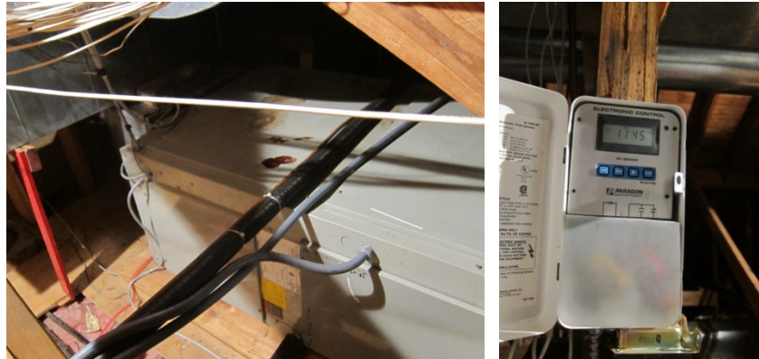
Air Handling Unit in Attic (L); Time Clock for AHU in Attic (R)
