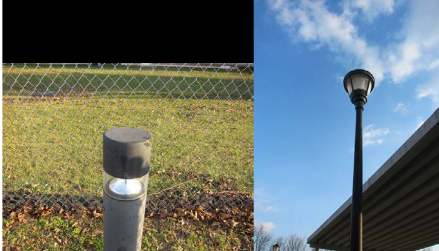
Typical CFL bollard and pole mounted mercury vapor fixtures
