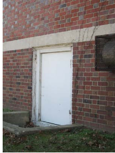
Signs of moisture in the brick façade and ground vegetation growing on wall (moisture in the wall)
