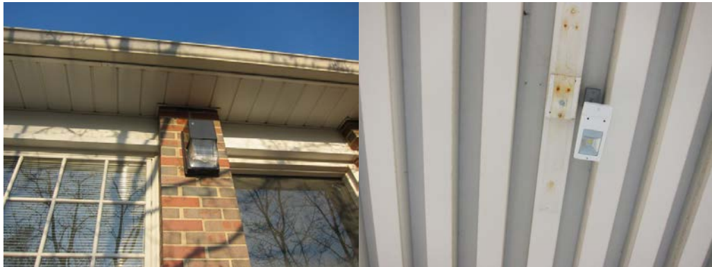
Typical metal halide and LED exterior fixtures
