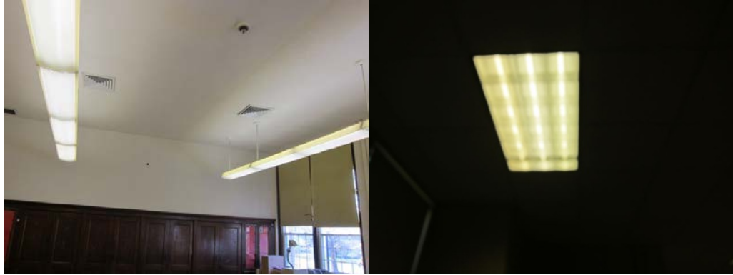
Typical interior T8 lighting in the old building (L.) classroom T8 lighting in the new building (R.)
