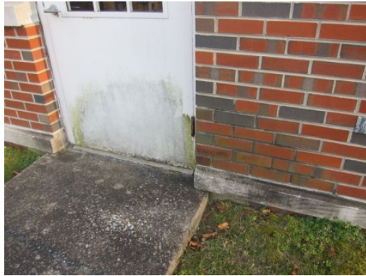
Signs of moisture in the brick façade and ground vegetation growing on wall (moisture in the wall)
