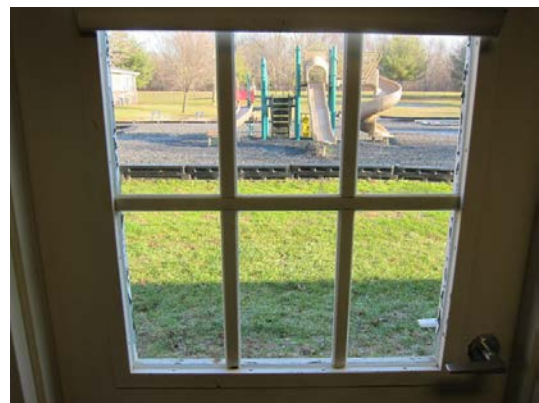
Typical exterior doors are non-insulated aluminum with single-pane glass panels
