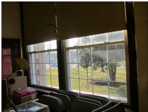
Typical single-hung type windows with clear double glazing and a non-insulated frame. Note: the green light on the low-E detector indicates clear glazing. (Old Building)
