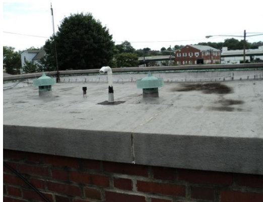
Typical bathroom exhaust fans
