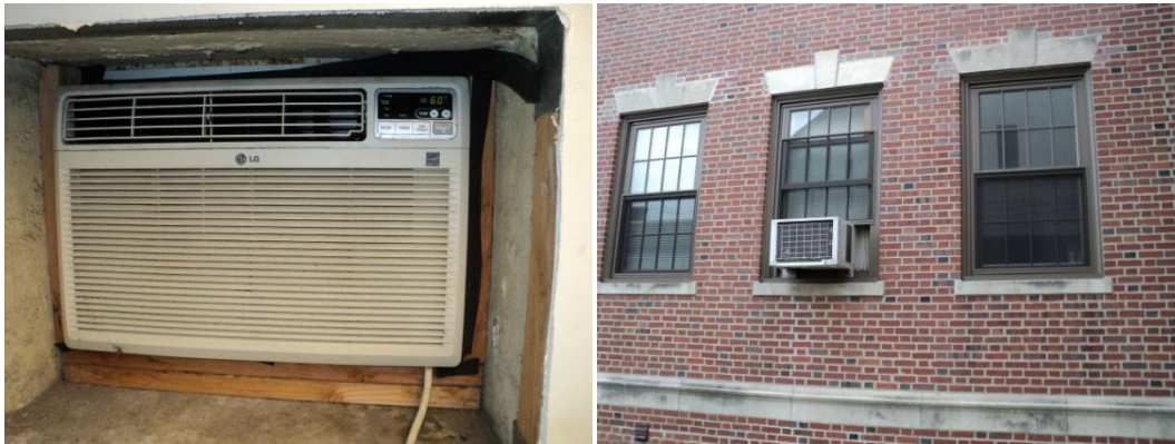
Typical through-the-window and through-the-wall air conditioners
