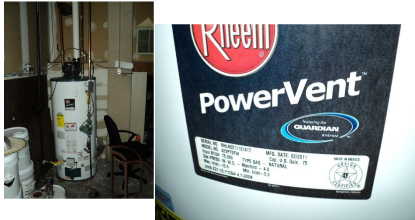
Existing Domestic Hot Water Heater and Nameplate
