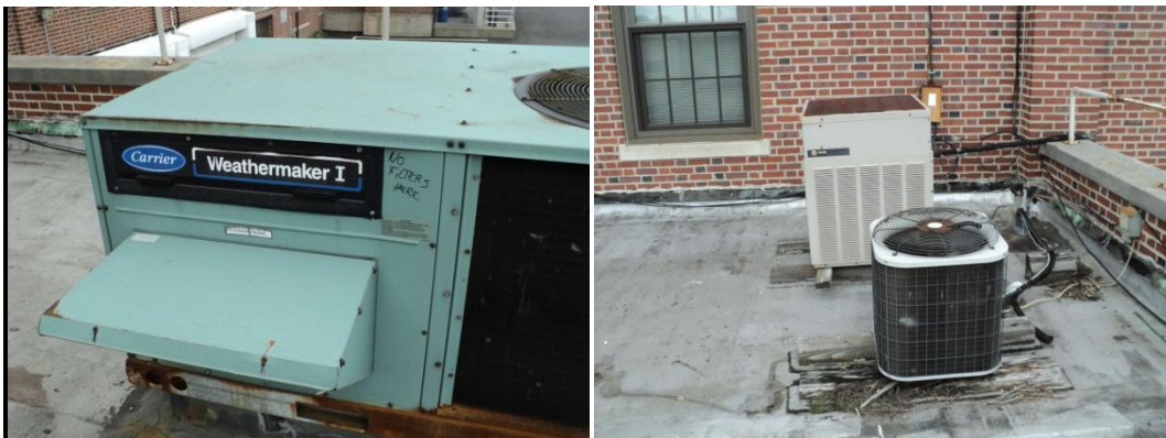
Existing Carrier Trane Split System and Carrier Heat Pump (R.)
