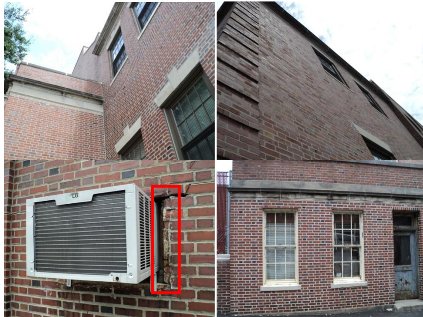
Typical exterior wall surfaces and cracked bricks and mortar joints and un-sealed exterior wall penetrations around through-the-wall air conditioners.
