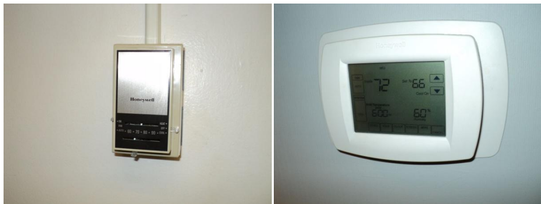
Typical manual (L.) and digital programmable thermostats (R.)
