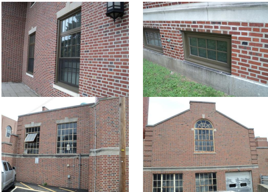
Typical installed windows with damaged window frames and single-glazed windows with ineffective frames
