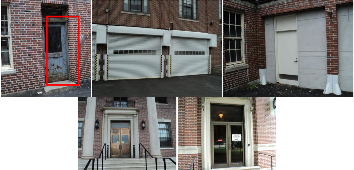
Typical exterior doors with damaged door to boiler room section.
