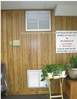
Wall mounted return grills for AHU-3 in Court Rm (left); Air intake control dial (middle); Duct installed damper on outside air intake for AHU-3 (right)
