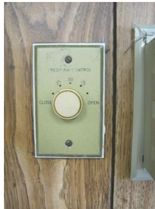
Wall mounted return grills for AHU-3 in Court Rm (left); Air intake control dial (middle); Duct installed damper on outside air intake for AHU-3 (right)
