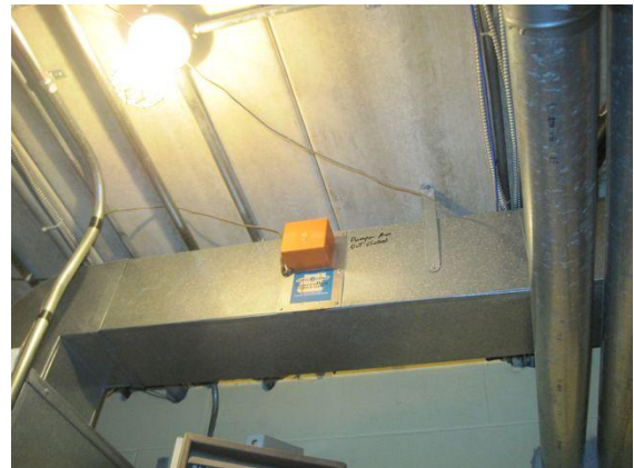
Wall mounted return grills for AHU-3 in Court Rm (left); Air intake control dial (middle); Duct installed damper on outside air intake for AHU-3 (right)
