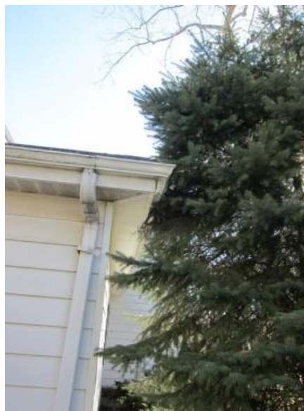
Ground vegetation touching/overhanging roof surfaces, and broken branches can lead to clogged drains
