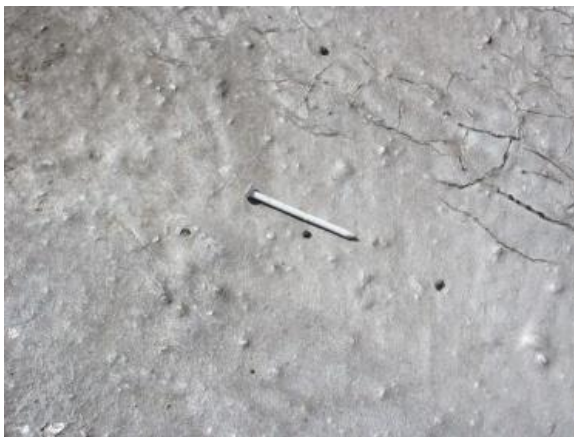
Rocks/nails or other sharp objects on roof surface, and debris including small CO2 cartridges
