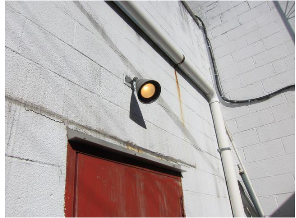
Exterior flood lights. Note the light on the right (on fire station) is illuminated during daytime
