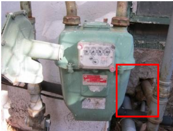
Un-caulked/un-sealed exterior wall penetrations
