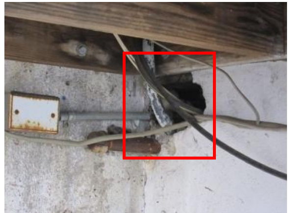
Un-caulked/un-sealed exterior wall penetrations
