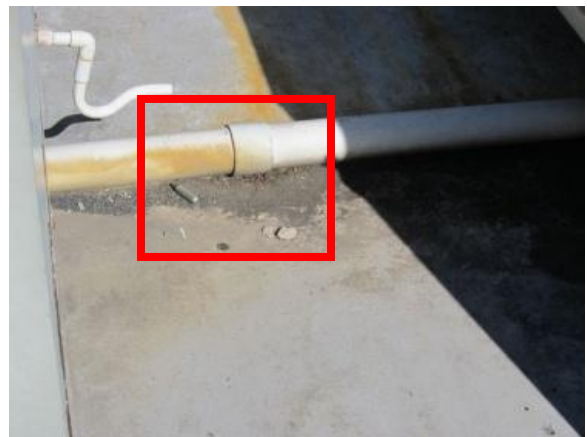
Rocks/nails or other sharp objects on roof surface, and debris including small CO2 cartridges
