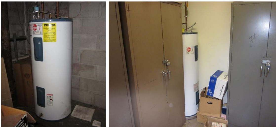
Police Department and Senior Center DHW – excellent condition
