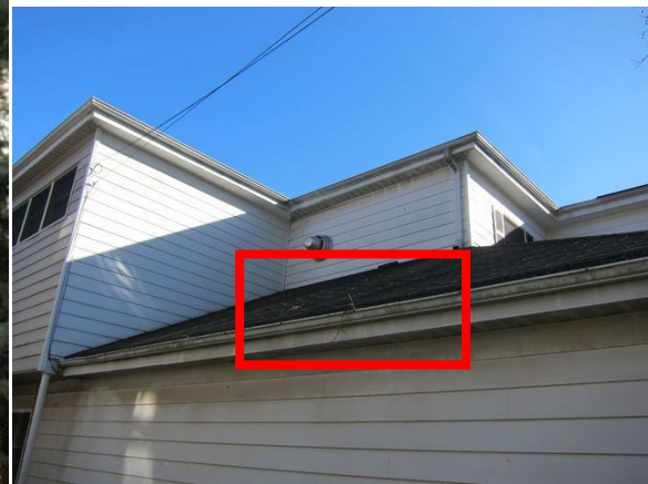
Ground vegetation touching/overhanging roof surfaces, and broken branches can lead to clogged drains
