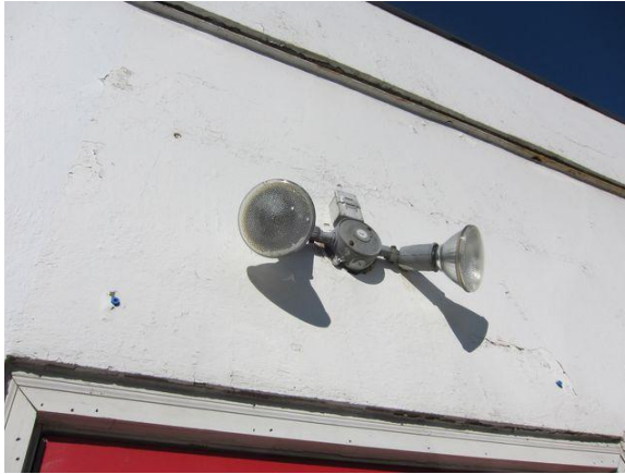
Exterior flood lights. Note the light on the right (on fire station) is illuminated during daytime
