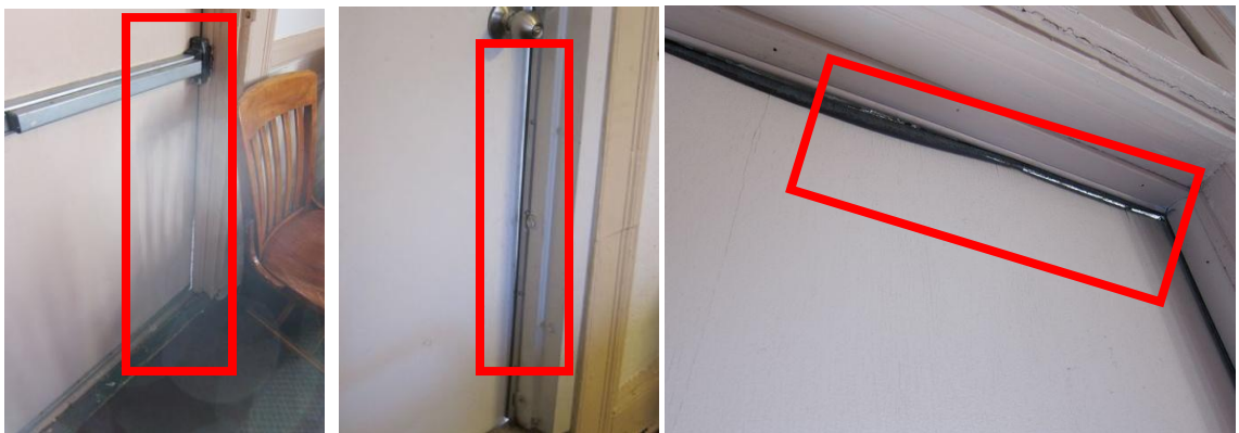
Missing/worn weather-stripping
