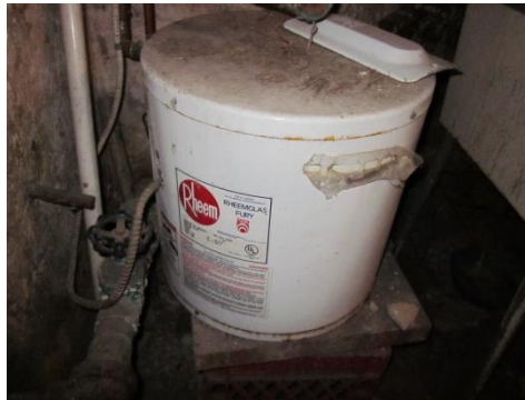
Rheem electric DHW heater
