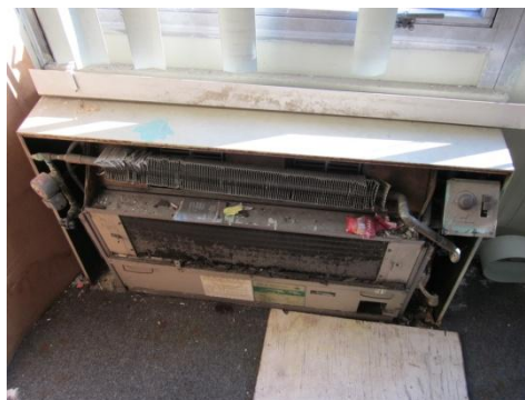
Unit ventilator in Classroom Level-4
