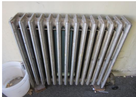
Cast iron steam radiator on 2 nd floor
