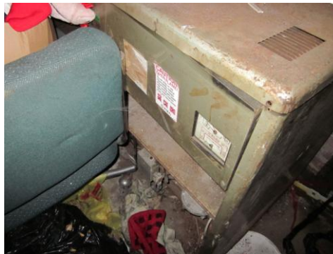
Unused boiler that should be removed
