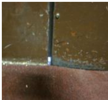
Worn/ Missing Weather-stripping
