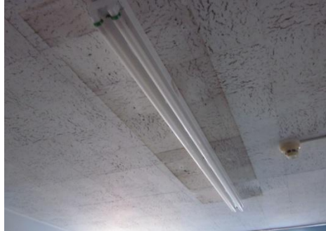
Typical T12 fixture with magnetic ballast
