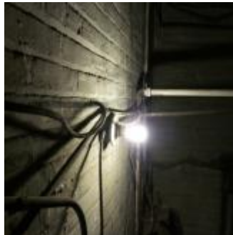
Un-insulated brick façade
