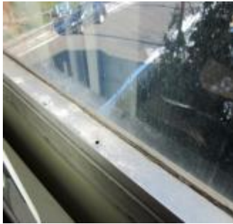
Single-glazed window with ineffective frame
