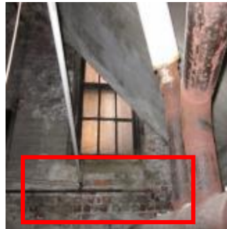
Cracked/deteriorated bricks and mortar joints
