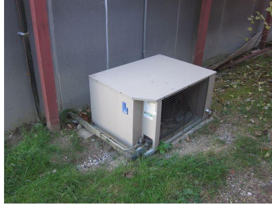
Walk in Freezer Cooler (left) and Freezer Condensing unit outside (right)
