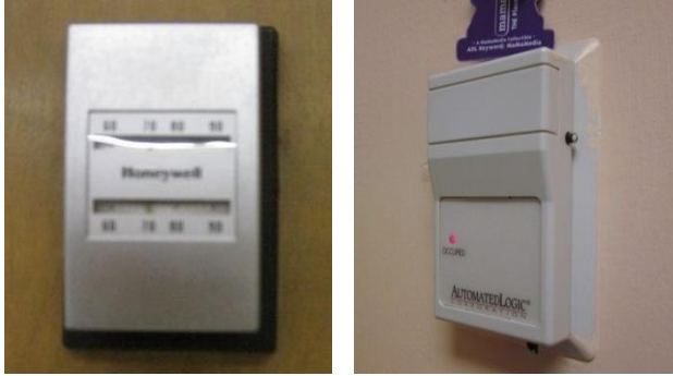
Manual thermostats for Unit Ventilators, Typical; Programmable thermostat for Annex RTUs
