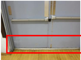
Missing/worn weather-stripping
