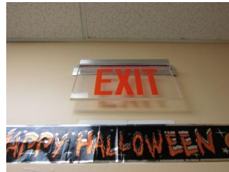
Incandescent exit signs were found in older parts of the building, while LED exit signs were found in the Annex
