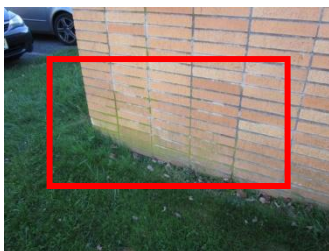
Signs of uncontrolled roof water runoff on walls due to missing/defective roof flashing
