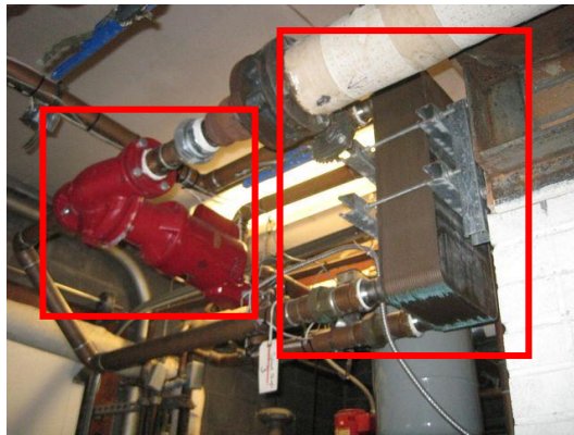
Plate and Frame Heat Exchanger & Pump; Heat Exchanger Piped to Hot Water header
