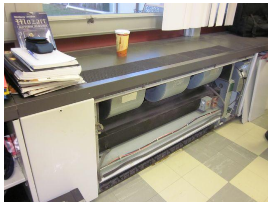
Trane Unit Ventilator, Typical D Wing; McQuay Unit Ventilator, Typical
