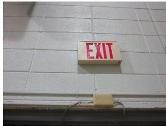
Incandescent exit signs were found in older parts of the building, while LED exit signs were found in the Annex
