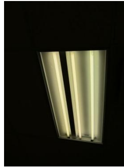
T8 linear fluorescent fixtures seen in the hallways, classrooms and offices
