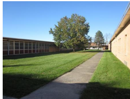
Partial Right Side Façade Courtyard
