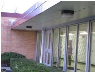
Metal Halide fixtures seen throughout the exterior of the building
