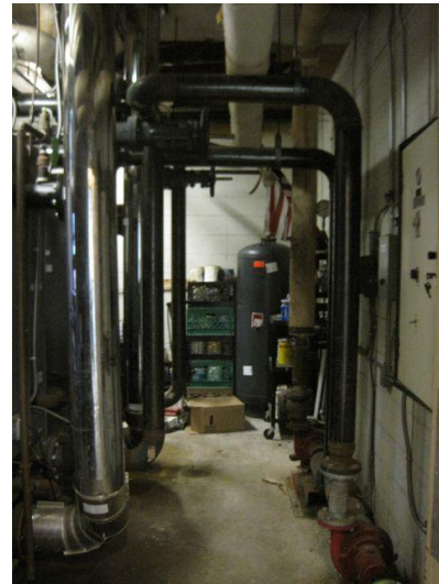
Aerco 200 MBTU Condensing Boilers; Stainless Steel Flue Piping
