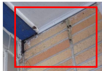
Insect nesting in exterior wall cracks and cavities
