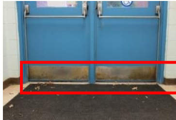
Missing/worn weather-stripping
