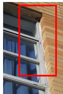
Cracked or aged caulk around frame/sill on the exterior
