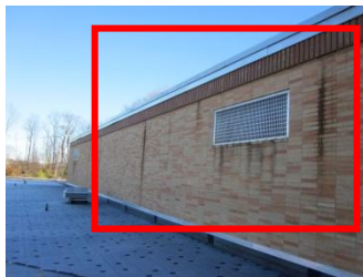
Signs of water damage at perimeter walls due to missing/ineffective site drainage
