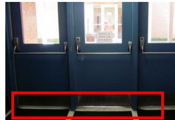
Missing/worn weather-stripping
