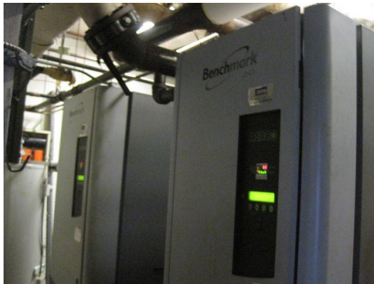
Aerco 200 MBTU Condensing Boilers; Stainless Steel Flue Piping
