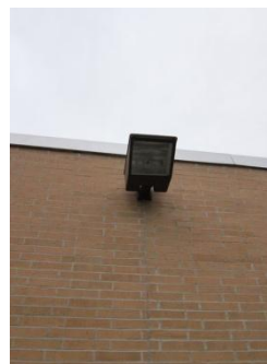
Metal Halide fixtures seen throughout the exterior of the building
