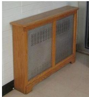
Cabinet Unit Heater at Building Entrance
