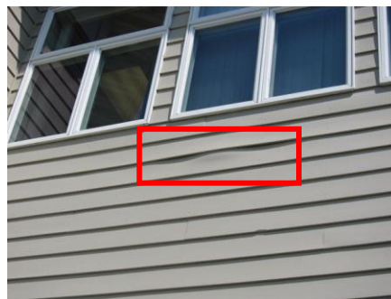
Warped siding
