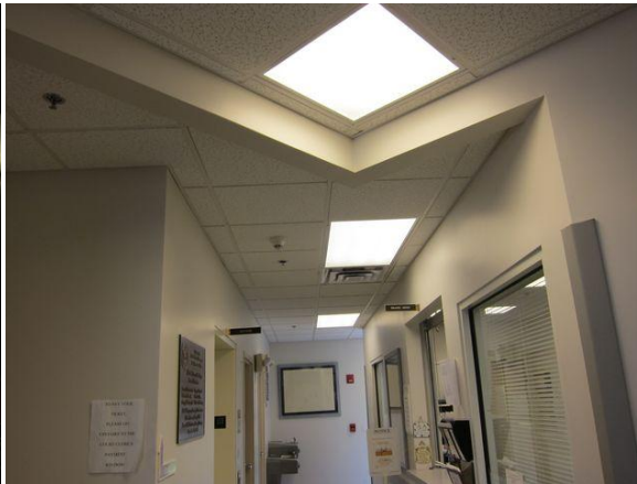
Typical T8 and recessed halogen fixtures
