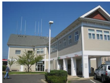
South-East Façade and Rear Entrance
