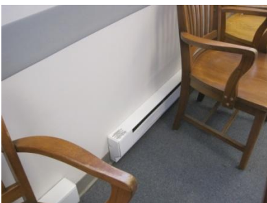
Typical baseboard electric unit heaters; Unit heater temperature control knob (right)
