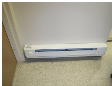
Typical baseboard electric unit heaters; Unit heater temperature control knob (right)
