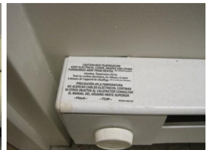
Typical baseboard electric unit heaters; Unit heater temperature control knob (right)
