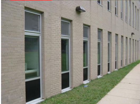
Exterior water damage signs on areas around windows and ineffective drip-edge detail
