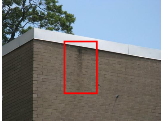
Typical exterior wall surfaces with signs of cracked bricks and mortar joints, damaged exterior wall finishes, and water damage.
