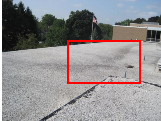
Typical roof surfaces with signs of water pooling and water damage
