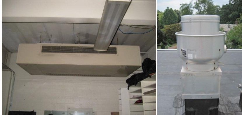
Typical unit ventilators and exhaust fans
