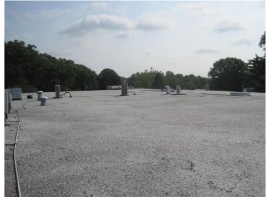
Typical roof surfaces with signs of water pooling and water damage
