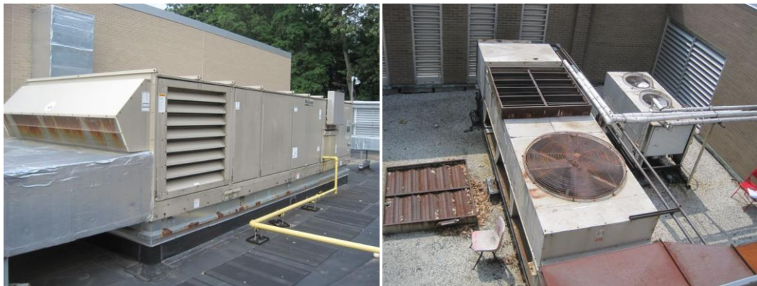
Typical rooftop packaged heating and cooling units.
