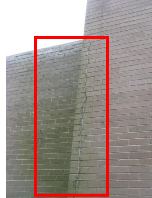
Typical exterior wall surfaces with signs of cracked bricks and mortar joints, damaged exterior wall finishes, and water damage.
