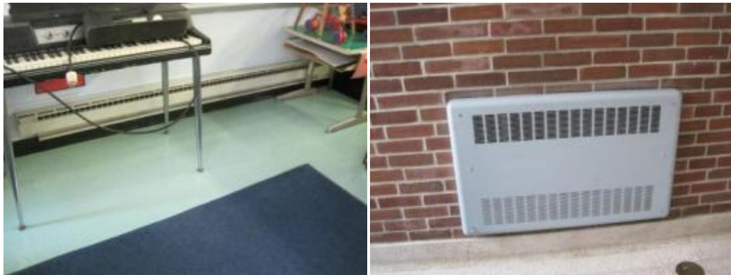
Electric Radiators in Wing classrooms; Wall Mounted steam radiators
