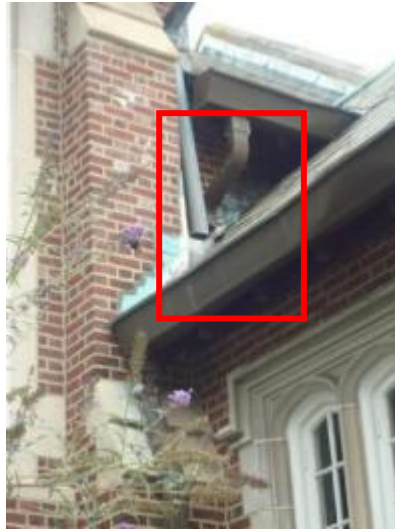
Missing drain pipe leading to 1st floor gutter
