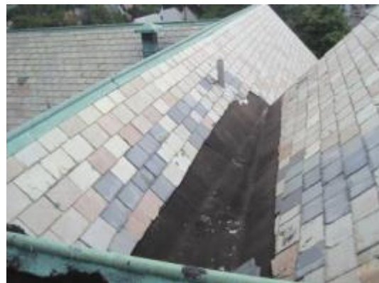
Missing roof shingles & Copper Trim oxidizing, leading to deterioration
