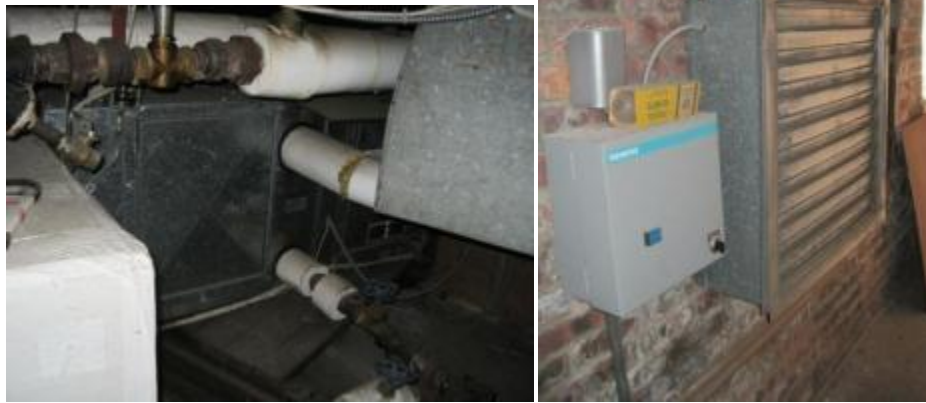
Library AHU in attic; Attic exhaust fan with Siemens control
