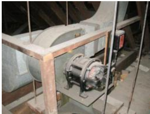
Abandoned exhaust fan in Main Attic
