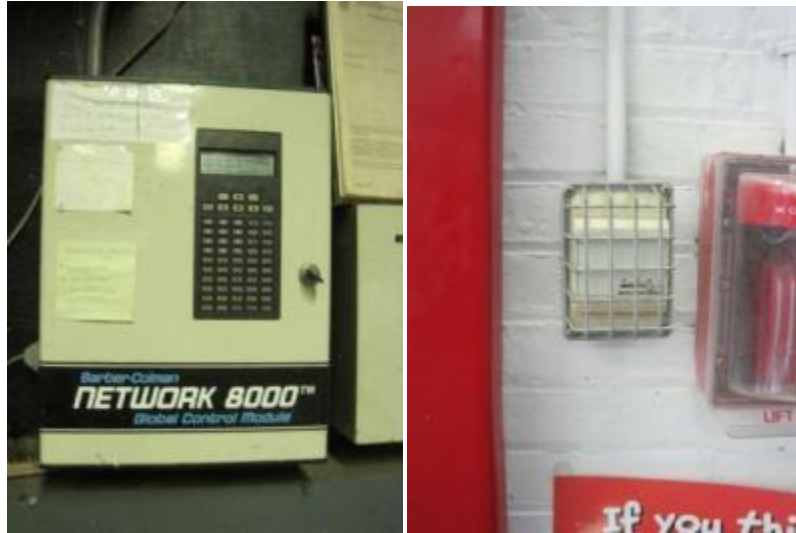
Barber Coleman controller; Gymnasium AHU thermostat
