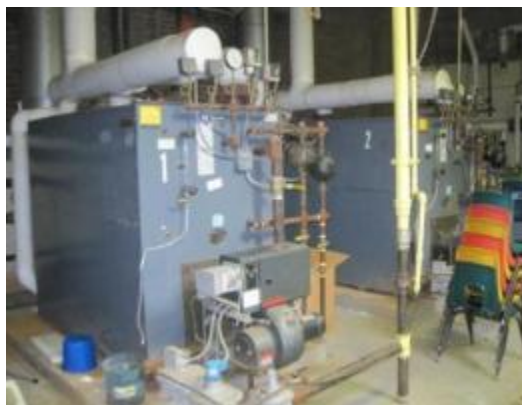
Cast Iron Steam Boilers
