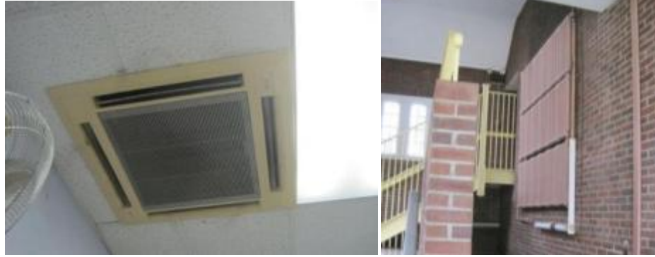
SF-1 OA intake and heater for Main Office; stairwell steam radiator
