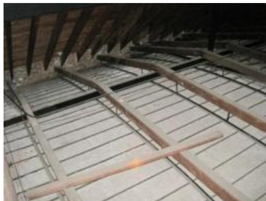
No insulation above ceiling
