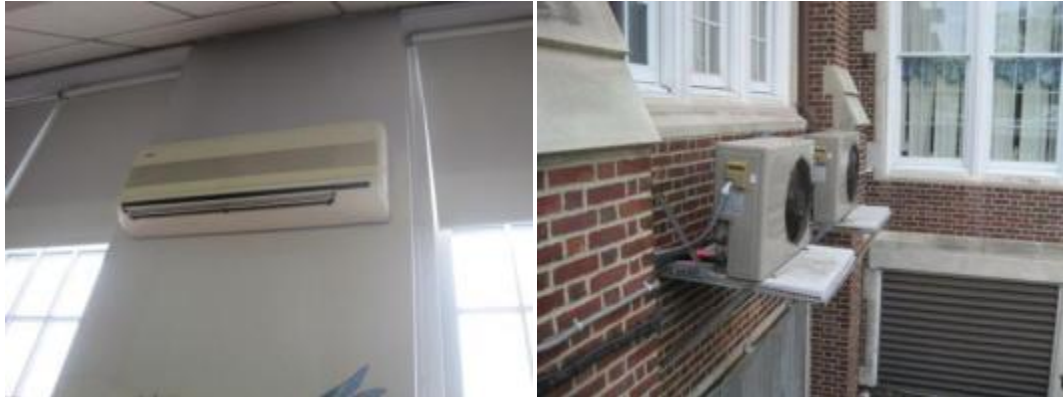
Wall Mounted DX Split System Indoor Unit and Outdoor Condensers
