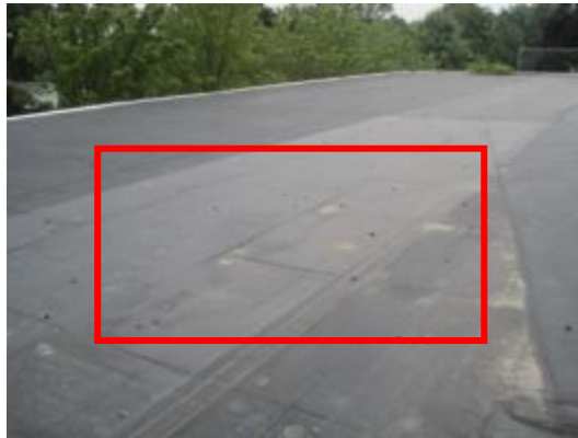
Rocks/nails or other sharp objects on roof surface on Wing flat roof
