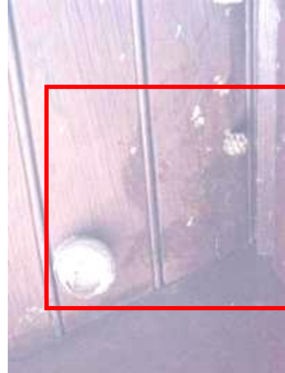
Insect nesting in exterior wall cracks and cavities
