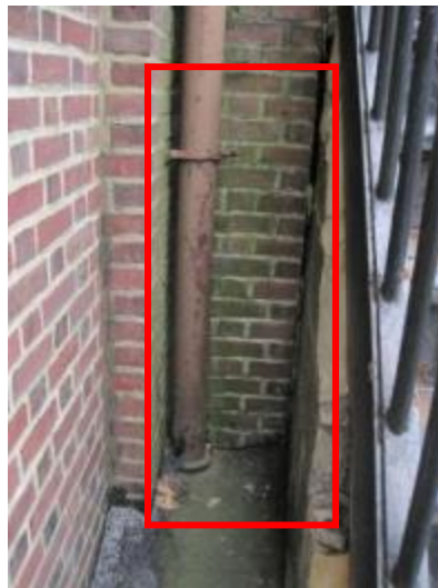
Signs of water damage at perimeter walls due to ineffective site drainage
