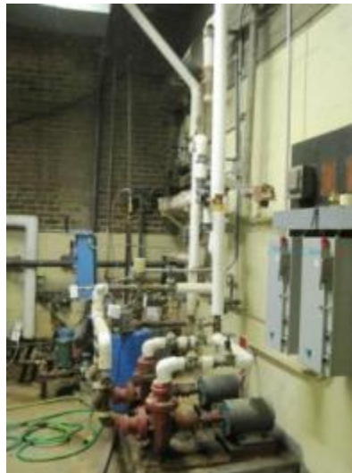
Hot Water Distribution to Wing
