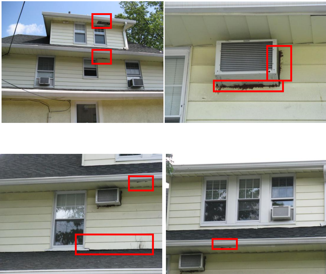
Typical exterior wall systems with missing siding and damaged exterior wall finishes; as well as damage around an improperly sealed and insulated exterior wall penetration.
