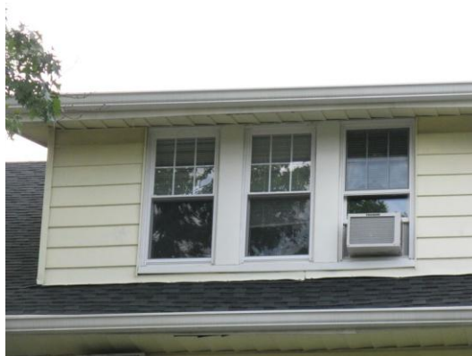
Typical window units with air-leakage at sleeved window conditioning units
