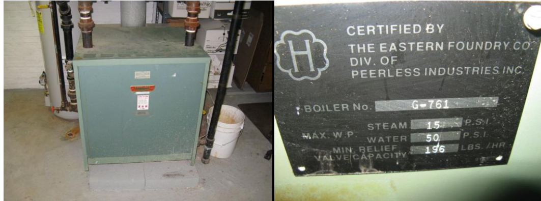
Existing Peerless boiler and nameplate
