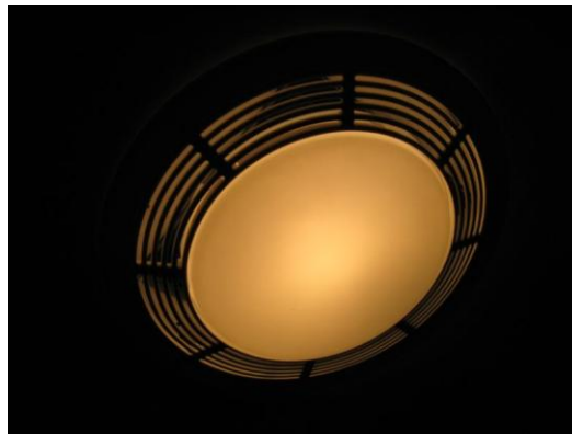
Typical combination exhaust fans and bathroom light units.
