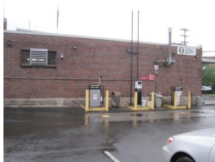
South-East Facing Façade
