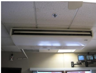
Dispatch air handler/evaporator
