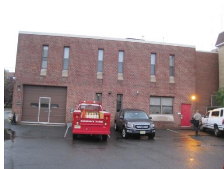
South Facing Façade, Rear Entrance
