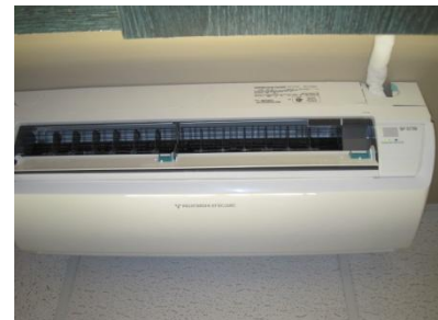
Kitchen air handler/evaporator
