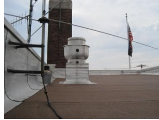
Pitched asphalt roof
