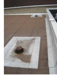
Cleared roof drains
