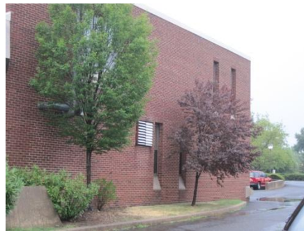
West Facing Façade
