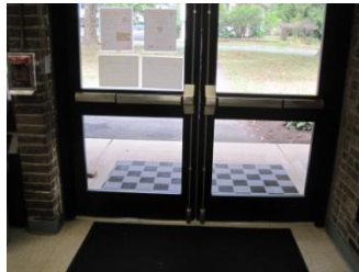
Missing/worn weather-stripping
