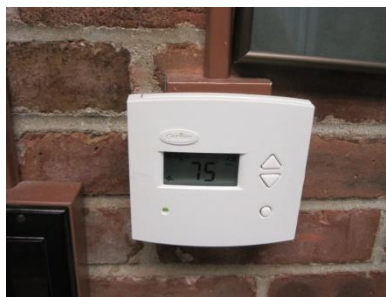
Typical: Programmable thermostats for cooling;
