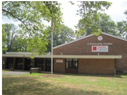
North West Façade and Main Entrance
