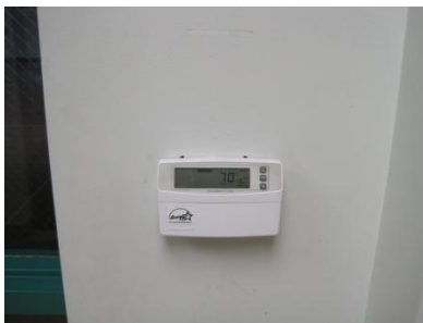
Typical: Programmable thermostats for cooling;
