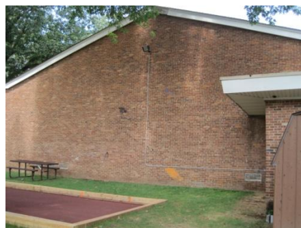
South East Façade and Rear Façade
