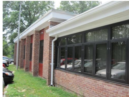
North East Façade
