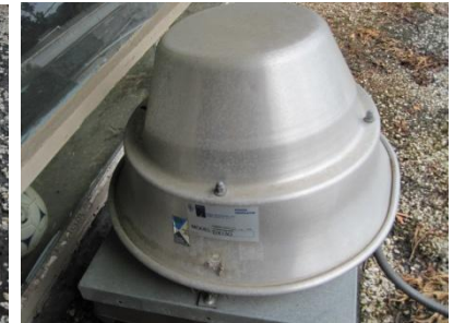
Two bathroom inoperable exhaust fans
