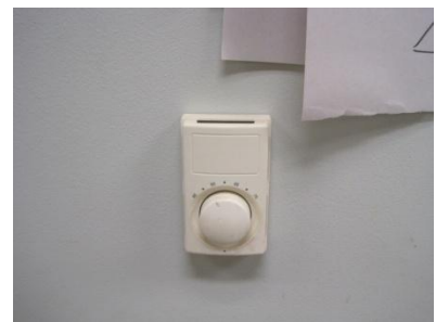
Manual thermostat for heating
