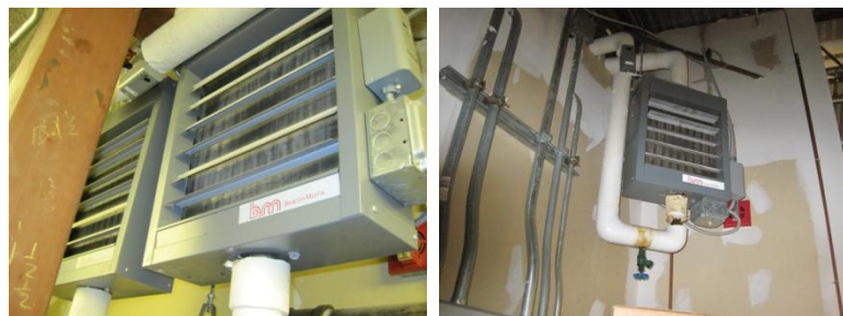
Ceiling hung hydronic heaters (typical)
