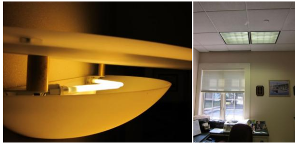
Compact Fluorescent scone fixture and typical T12 fixture
