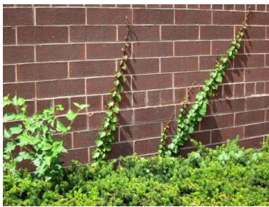
Overgrown ground vegetation touching/blocking exterior wall surfaces
