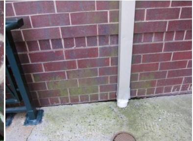
Uncontrolled water run-off due to poor downspout seal
