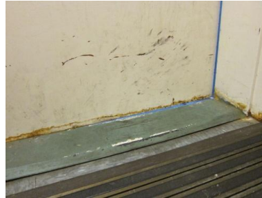
Missing/worn weather-stripping close-up of picture on left
