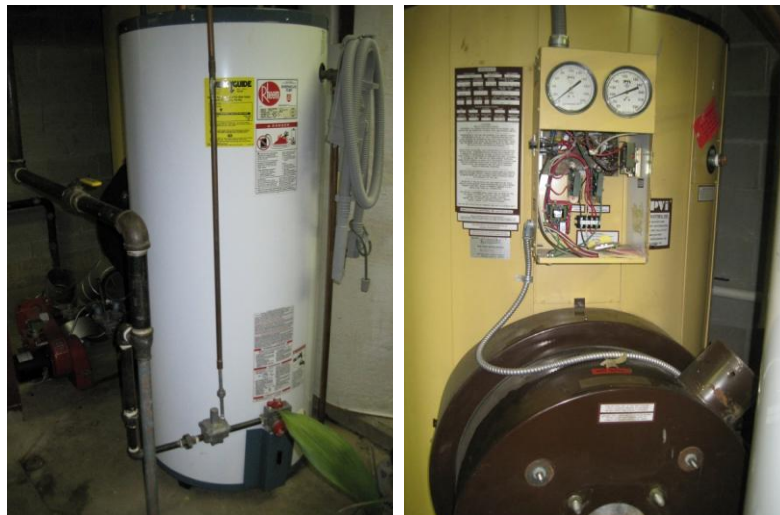
Rheem 100 gal storage replaces PVI 300 gal storage DHW
