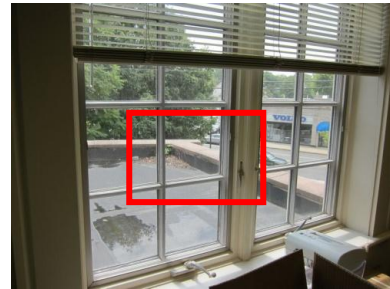
Uncontrolled vegetation growth on roof
