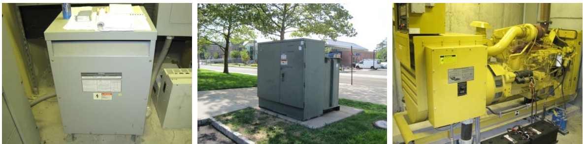
Siemens step-down/up transformer (typical); Main incoming transformer; Caterpillar emergency generator
