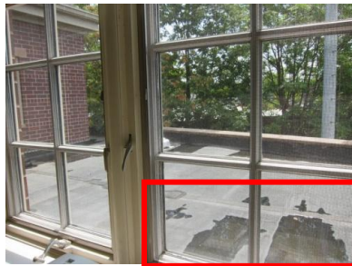
Signs of standing water/pooling
