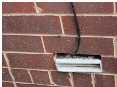
Un-caulked/un-sealed exterior wall penetrations
