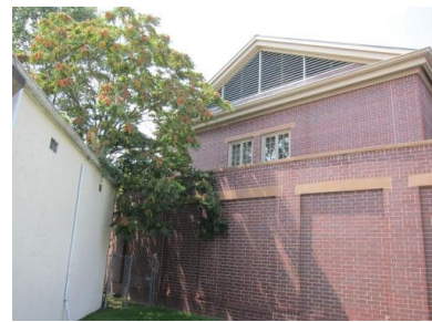
Overgrown ground vegetation touching/blocking exterior wall surfaces
