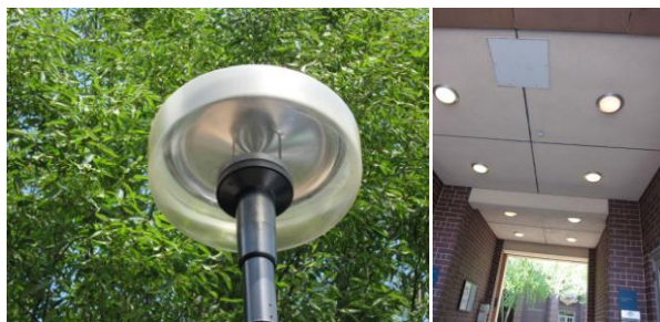
Pole mounted Metal Halide parking lot and recessed exterior fixtures
