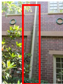
Uncontrolled roof water run-off due to defective/clogged gutters and downspouts
