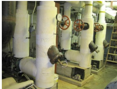
City Hall heating hot water circulators
