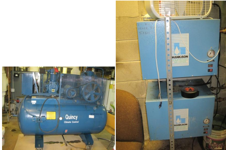
Instrument air compressor; Instrument air refrigerated dryer
