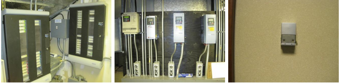
Typical: Input/output electronic to pneumatic signal panels; Fan VFDs; Area thermostat
