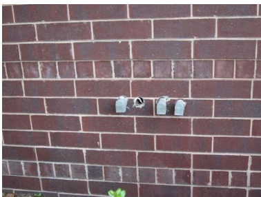
Un-caulked/un-sealed exterior wall penetrations
