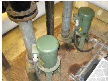
Lift station (typical)
