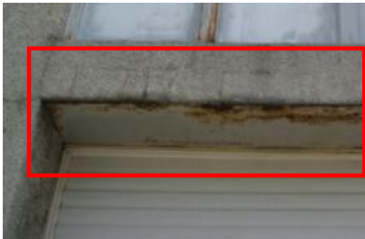
Exterior mold/water damage signs on areas around doors
