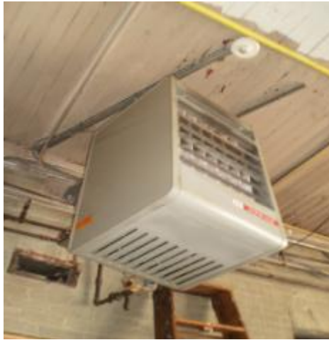
Typical convective unit heater in garage
