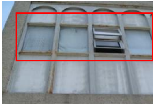
Exterior mold/water damage signs on areas around windows
