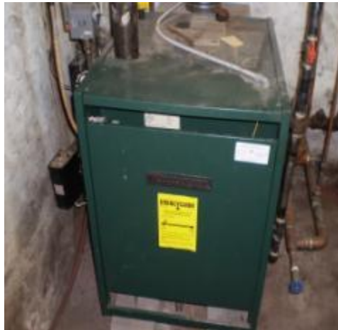
Williamson steam boiler with un-insulated pipe
