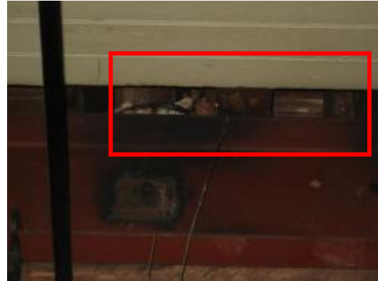
Missing attic insulation between wooden rafters
