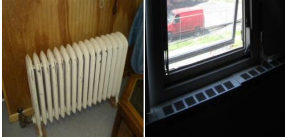
Steam radiator (L); Electric baseboard under window (R)
