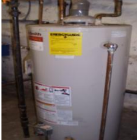
Atmospheric DHW heater
