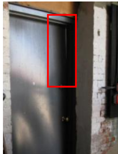
Missing/worn weather-stripping
