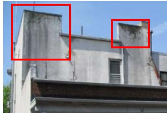
Signs of water damage at perimeter walls due to missing/ineffective site drainage
