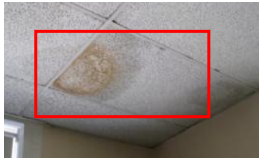
Sagging/water damaged ceiling tiles in many areas due to roof leaks
