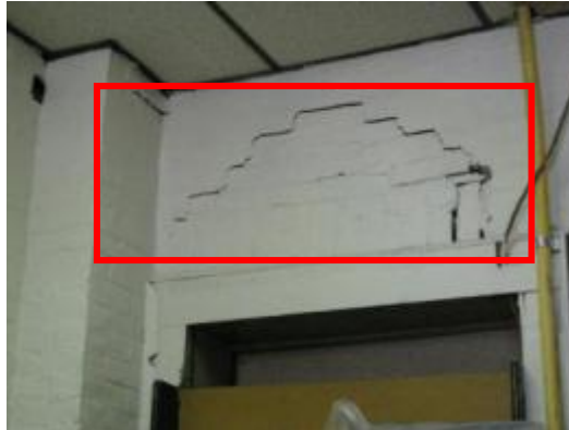
Cracked/deteriorated mortar joints; potential structural damage
