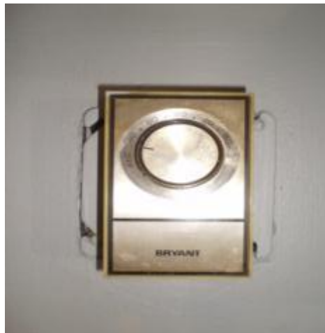
Bryant thermostat for electric heaters
