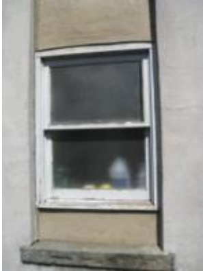
Missing/ineffectively-applied caulk around frame or sill on the exterior
