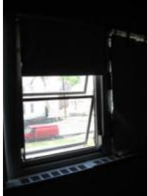
Single-glazed window with ineffective frame
