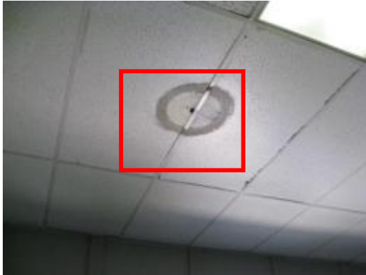
Sagging/water damaged ceiling tiles in many areas due to roof leaks
