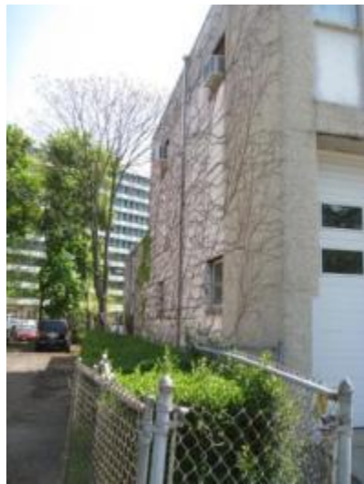
Overgrown ground vegetation covering exterior wall surfaces
