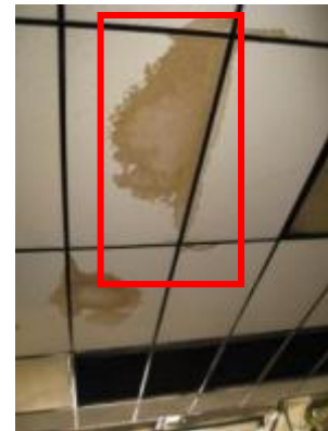
Sagging/water damaged ceiling tiles in many areas due to roof leaks
