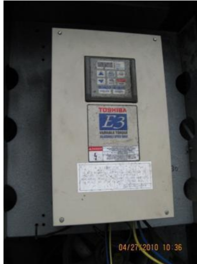
Toshiba VFD on RTU supply fan, typ.
