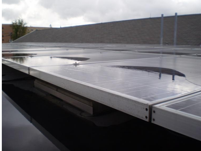
Standing water on flat-mounted solar panels
