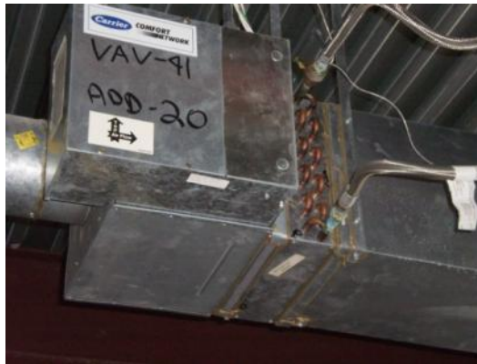
Typical VAV box with reheat coil connection
