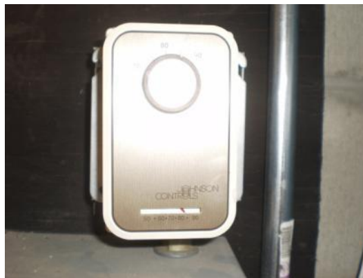
Hot water Unit heater thermostat, typ.
