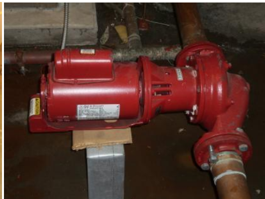
Hot water circulation pumps P-1 and P-2 standby; Hot Water booster pump mounted on cardboard
