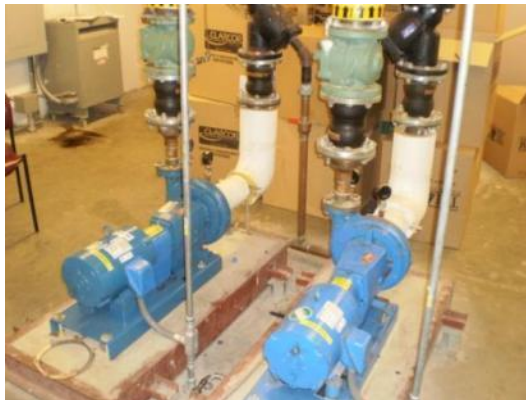
Hot water circulation pumps P-1 and P-2 standby; Hot Water booster pump mounted on cardboard
