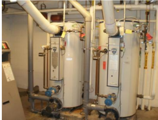
Condensing Domestic Hot Water Heaters
