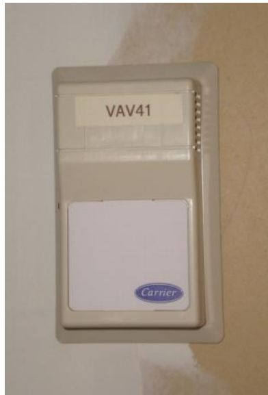
Typical VAV box temperature and humidity sensor
