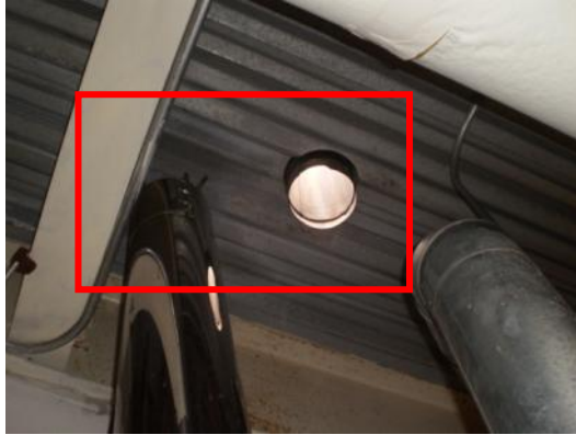
AO Smith flue pipe not connected to roof exhaust; Flue pipe damaged at base of boiler
