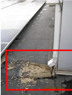
Deteriorated gutters pan
