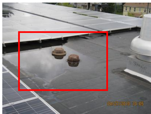
Signs of standing water due to raised drains
