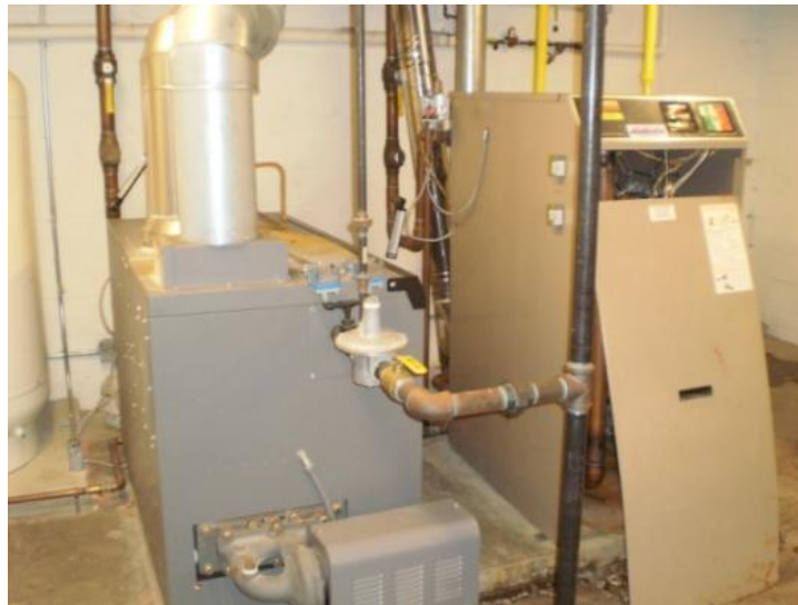
Laars boiler (left) and AO Smith boiler (right)
