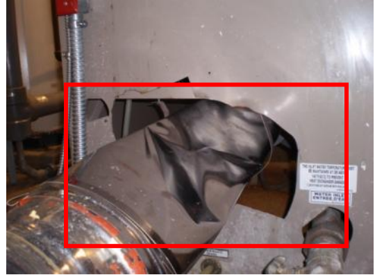
AO Smith flue pipe not connected to roof exhaust; Flue pipe damaged at base of boiler
