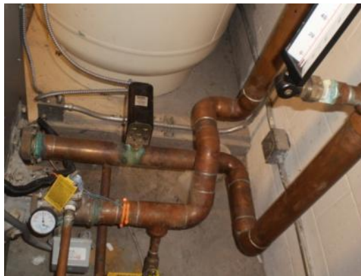
Missing insulation on hot water piping
