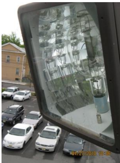
Exterior Metal Halide lights
