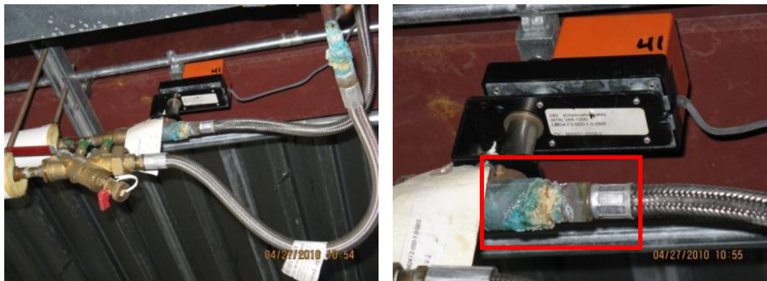
VAV Reheat automatic control valve; Corrosion that can cause leaks
