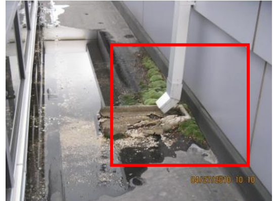
Uncontrolled vegetation growth on roof, on surfaces that do not have direct sunlight
