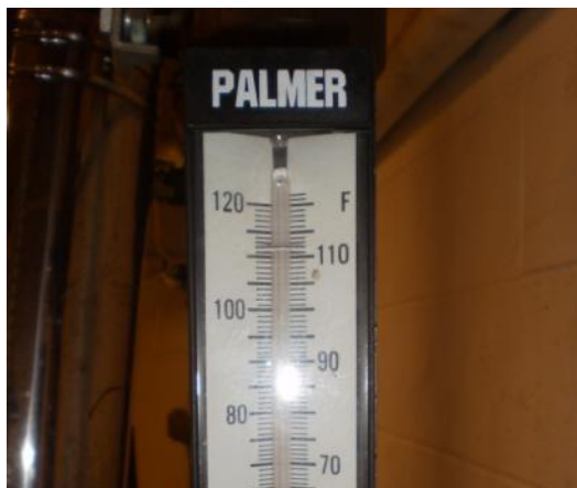
Thermostat at boiler supply with max temperature of 120°F
