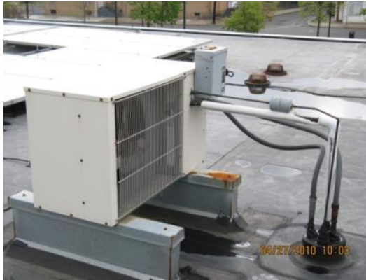
DX Split System Condenser on Roof with R-22 piping down to units on 1 st floor
