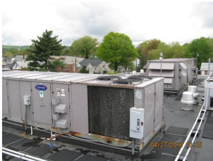
Carrier Rooftop Units RTU-2 & RTU-1
