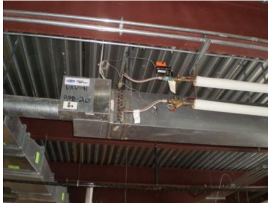
Typical Carrier VAV box with hot water reheat
