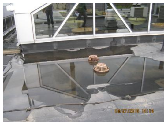
Signs of standing water due to raised drains
