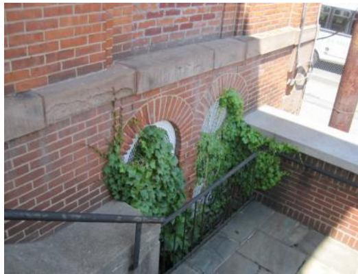
Overgrown ground vegetation touching/blocking exterior wall surfaces
