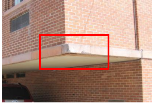
Damaged exterior wall finishes
