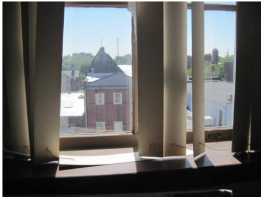
Single-glazed window with ineffective frame
