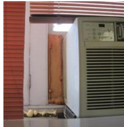
Air-leakage at sleeved window / wall air-conditioning units
