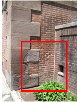
Cracked/deteriorated bricks and mortar joints
