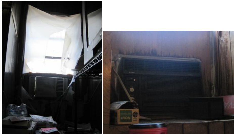
Aged Window AC Units in original section of building
