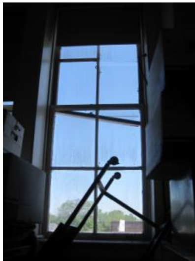
Damaged/aged window frame
