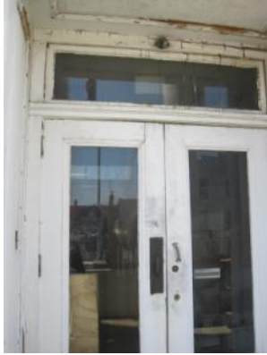
Damaged/warped/aged door frame
