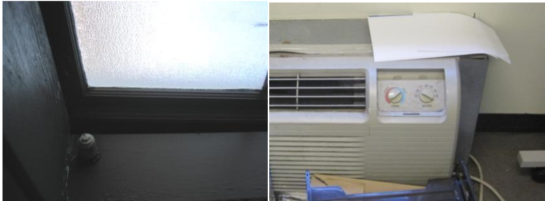
Steam radiator control dial (left); PTAC dial controls (right)
