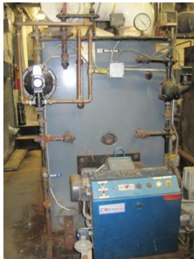
Operating Steam Boiler (left); Burnt Steam Boiler (right)
