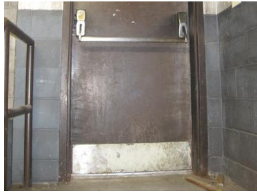
Missing/worn weather-stripping
