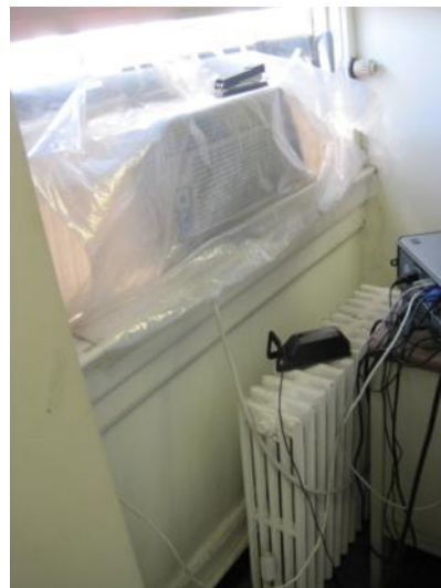
Steam radiator with enclosure (left); Exposed steam radiator below window AC (right)
