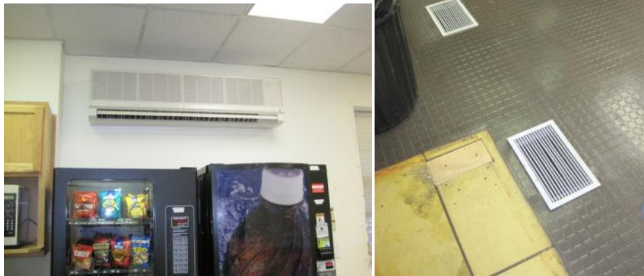
Sanyo wall mounted unit (left); Supply air diffusers (right)
