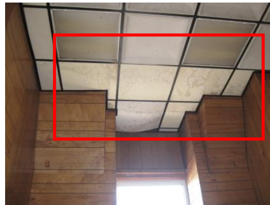
Signs of mold/water damage on interior finishes
