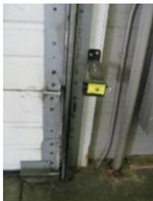
Missing/worn weather-stripping
