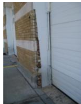
Damaged door frame
