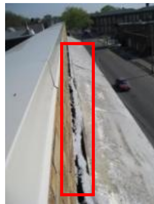
Eave is separating from exterior wall.
