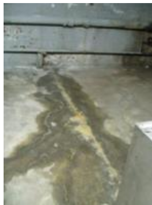
Water/moisture seepage through cracks detected in the slab
