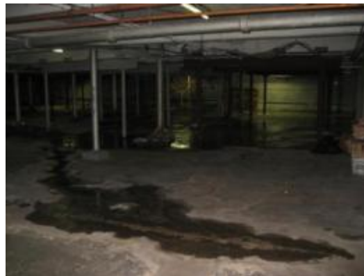
Water seepage from ground water
