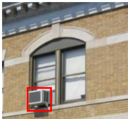
Air-leakage at sleeved window/wall air-conditioning units
