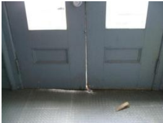
Aged wood type door with no weather stripping
