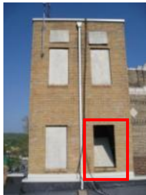
Open shaft on roof to 1st floor garage area, which brings in cold air. Only barrier is a poorly insulated door on the first floor.
