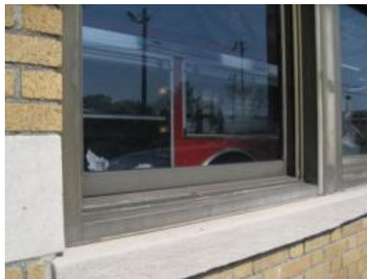
Single-glazed window with ineffective frame, difficult to open
