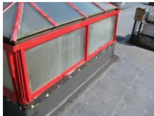
Single-glazed skylight, with ineffective frame
