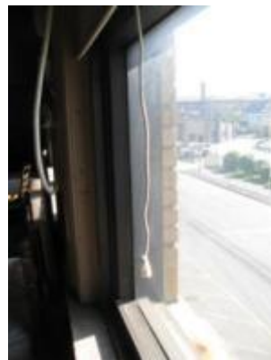
Single-glazed window with ineffective frame
