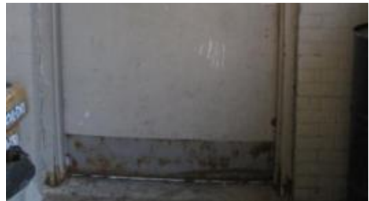
Missing weather-stripping on exterior door
