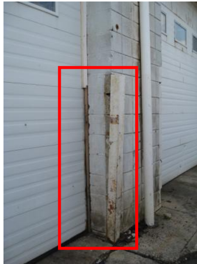
Severely damaged exterior wall trim/moldings
