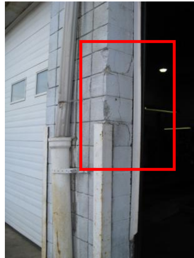
Substantial structural damage visible on exterior walls caused by water/ice build-up inside the envelope assembly
