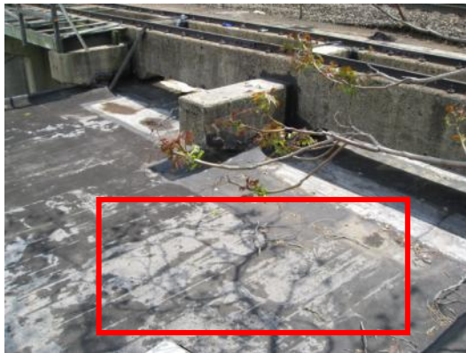
Membrane delamination, especially on lower section of roof.
