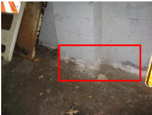
Deterioration at base of slab near salt storage area
