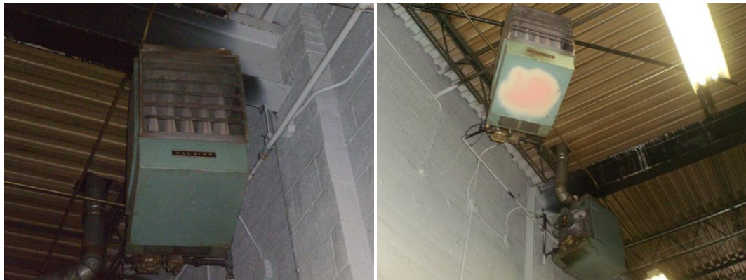
Carrier Gas Fired Unit Heaters
