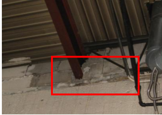
Signs of structural damage caused by water infiltration into roof cavity
