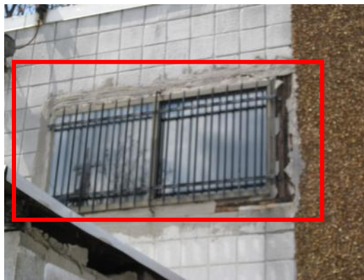
Severely cracked or aged caulk around frame/sill on the exterior
