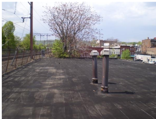
Rooftop bathroom exhaust fans
