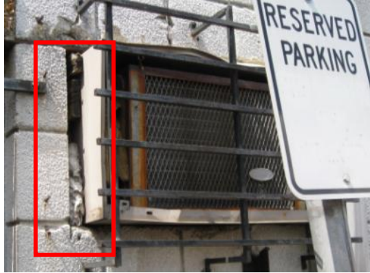
Poorly sealed exterior wall penetrations
