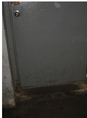
Typical door & Missing/worn weather-stripping
