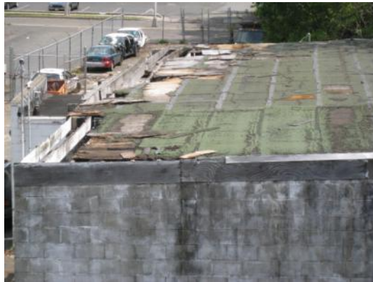
Severe roof deterioration
