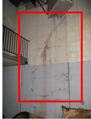
Substantial structural damage visible on walls caused by water/ice build-up inside the envelope assembly
