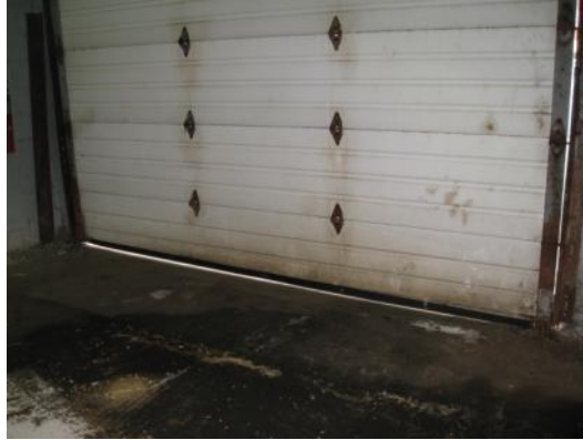
Missing/worn weather-stripping
