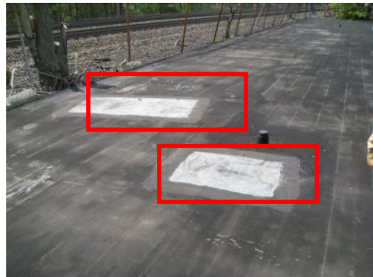
Delaminating roof membrane/patches.
