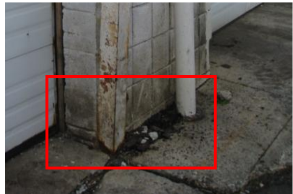
Deterioration at base of exterior slab
