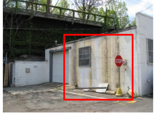
Severe damage to exterior wall due to uncontrolled water run-off
