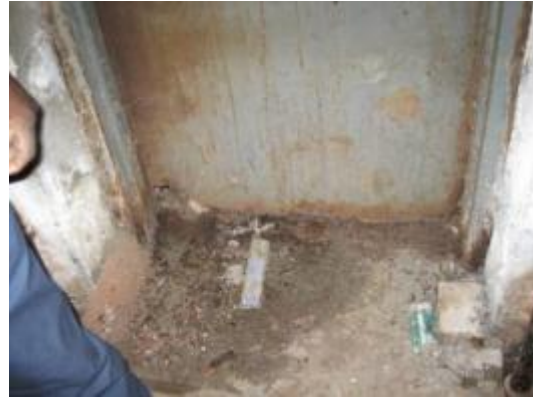
Water/moisture seepage through cracks detected in the slab
