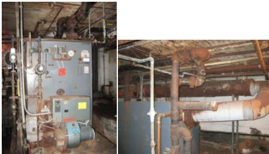
Weil McLain Natural Gas Steam Boiler; Rusty Piping and Flue, no insulation on piping
