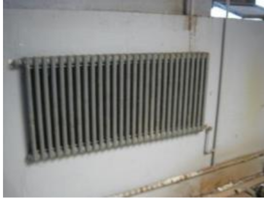
Steam Radiator Basement; Steam Fin tube Radiator Upper Floors
