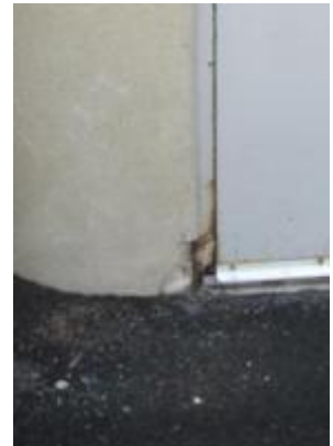
Damaged/warped/aged door frame
