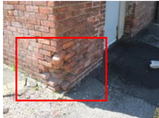
Cracked/deteriorated bricks and mortar joints
