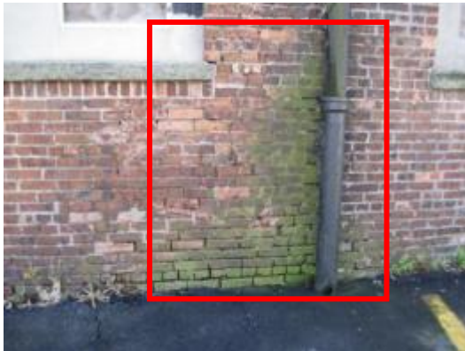
Signs of water damage and mold growth at perimeter walls due to missing/ineffective site drainage
