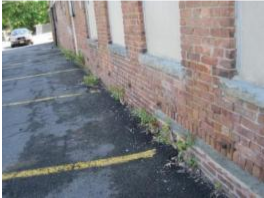
Structural cracks detected in the slab with vegetation growth
