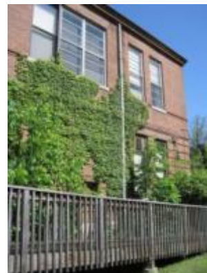
Overgrown ground vegetation blocking exterior wall surfaces
