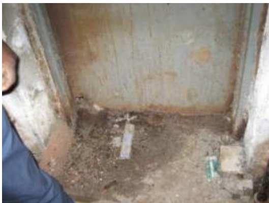
Interior mold/water damage signs on areas around doors
