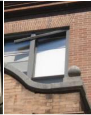
Damaged window frame
