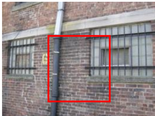
Cracked/deteriorated bricks and mortar joints
