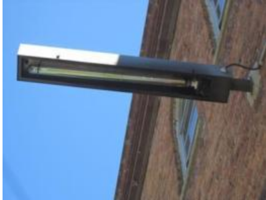
Exterior Metal Halide lights
