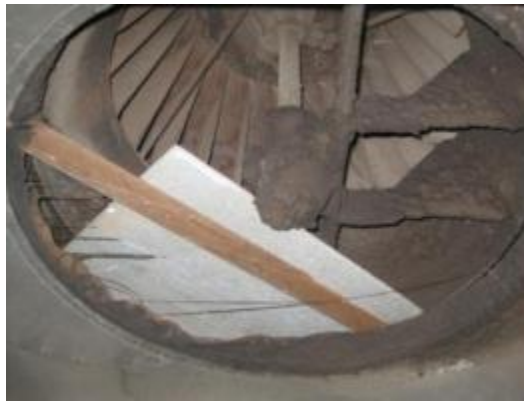
Abandoned Air Handling Unit; Blocked Outside Air Damper
