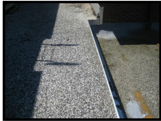
Tar and gravel roof.
