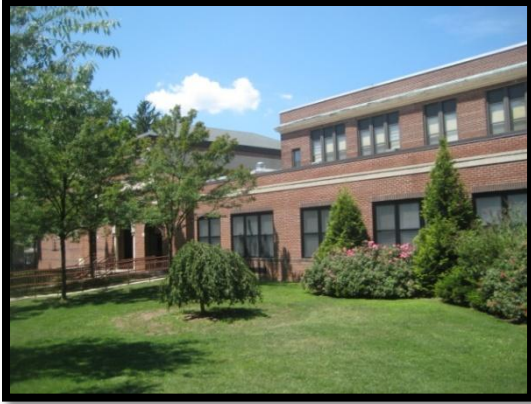
East Façade – Main Entrance
