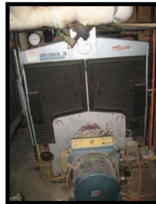
Gas-fired HW Boilers located in basement Boiler Room
