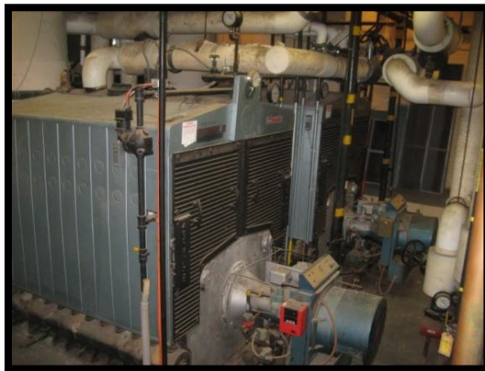
Gas-fired HW Boilers located in basement Boiler Room
