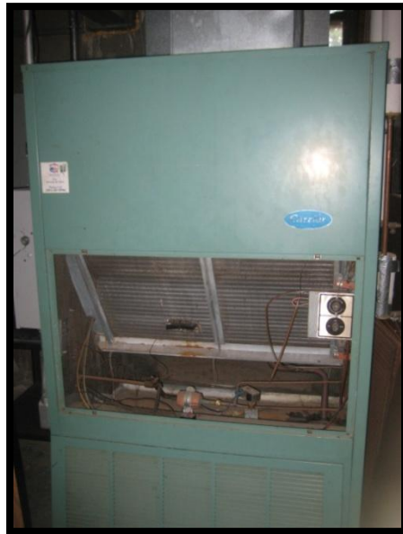
Outdated Carrier air handling unit with corresponding condenser.
