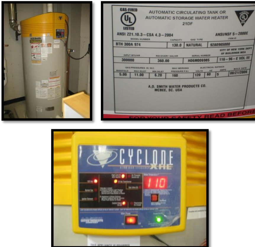
AO Smith gas-fired unit Domestic hot water heater
