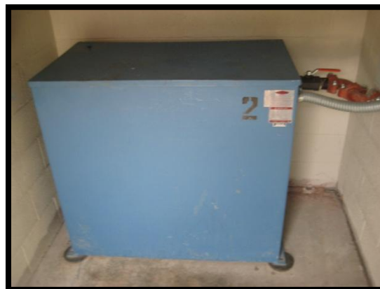
Hydraulic type elevator motor
