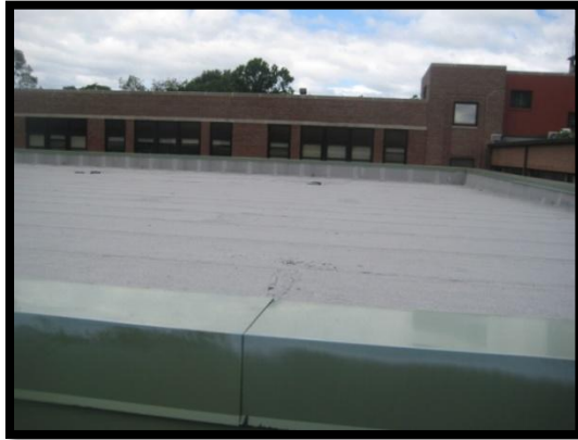
Flat asphalt roof
