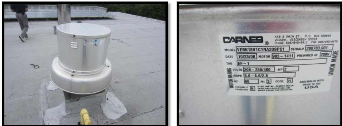
Typical rooftop exhaust fan unit
