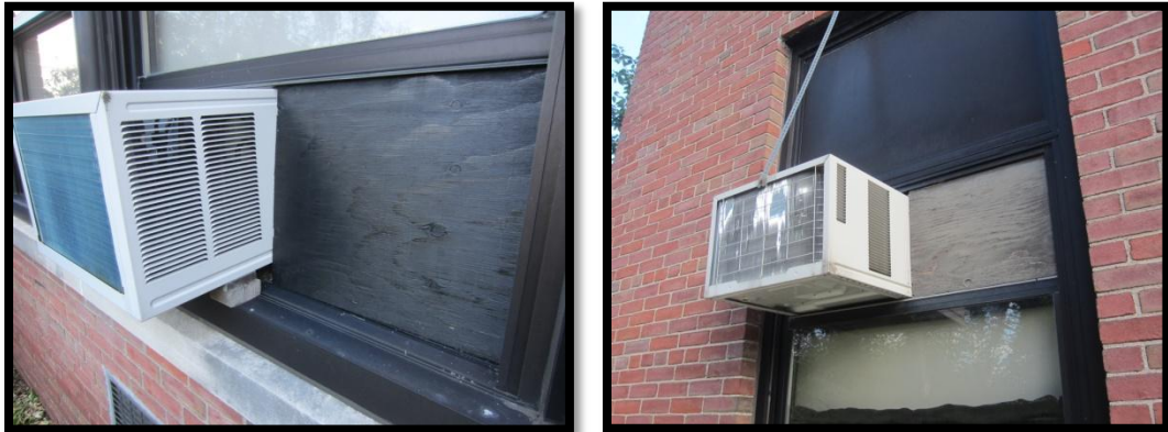
Window AC-Units sealed with a pieces of wood
