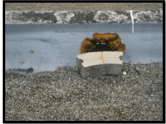
Deterioration on the base of roof parapet
