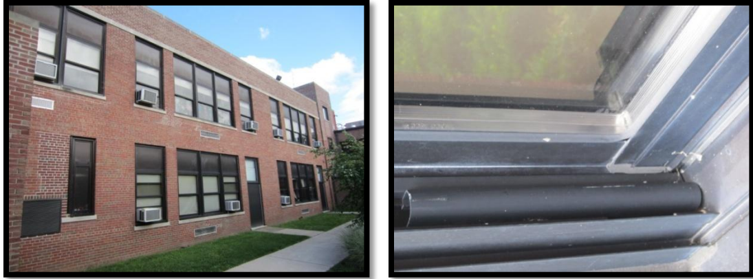
Typical double pane, aluminum frame windows. Units exhibit no signs of energy-compromising issues.
