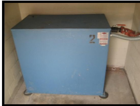
Hydraulic type elevator motor
