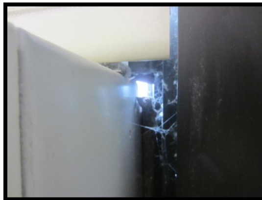
Gap of approximately 1in 2 around classroom window air conditioning unit
