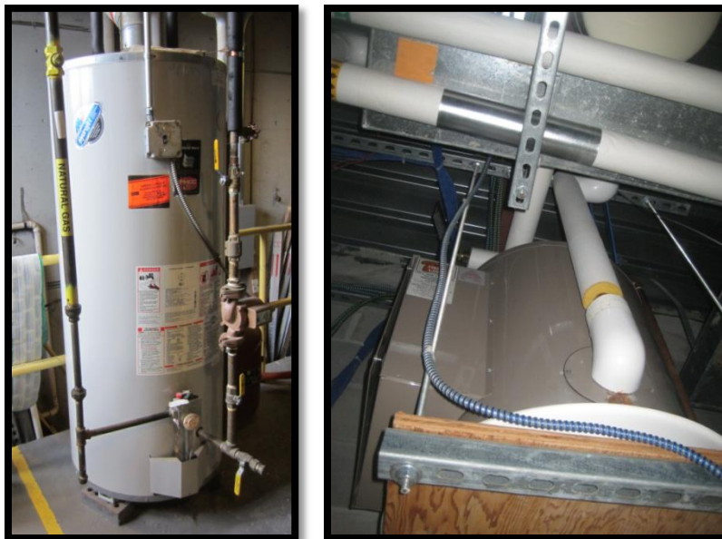
Bradford White gas-fired domestic hot water heater and electric water heater in "SSP" addition
