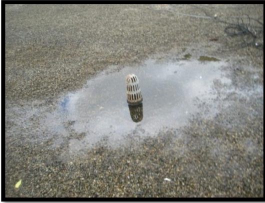
Ponding/standing water on roof
