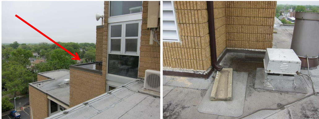
Dark-colored roof surface shows pooling water and effects cooling loads (L); pooling water near a down spout accelerates roof deterioration and may lead to leaking issues (R)
