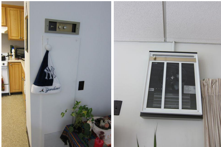
Typical fan coil unit found in apartment units (L) and typical electric wall heater (R)
