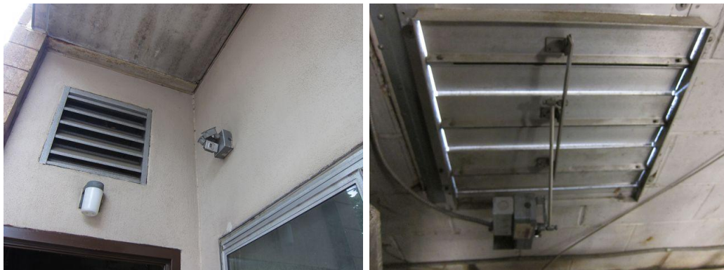
Emergency generator room louver is not mechanically controlled (L); mechanical outside air damper does not fully close when the hot water heaters are not operating (R)
