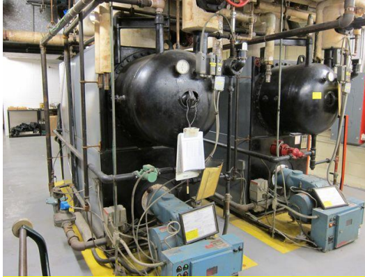
Thermo-Pak Heating Hot Water Boilers
