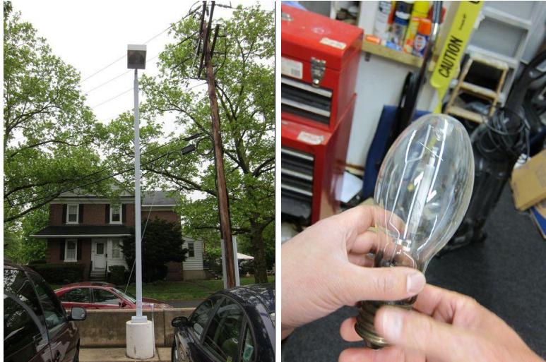
150 watt high pressure sodium parking lot lights
