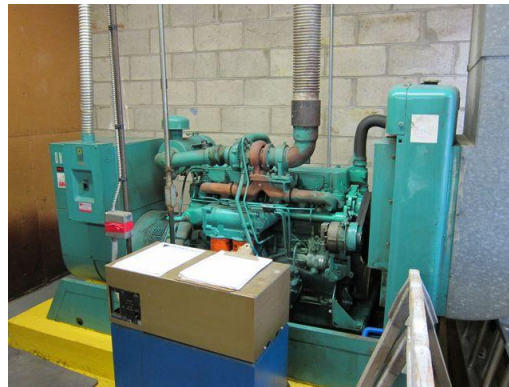
90 kW Onan emergency generator
