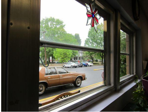
Clear single glazed window does not reduce solar radiation; the non-insulated aluminum frame acts as a thermal bridge
