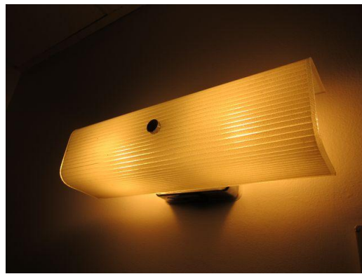
Typical recessed T8 lighting fixture (L); and wall mounted incandescent lamped fixture (R)
