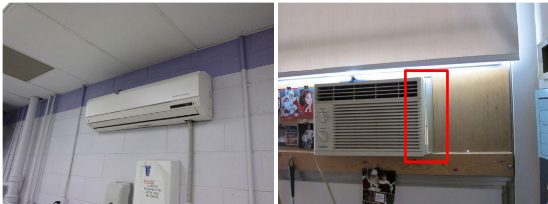
Typical split-DX indoor unit (L) and typical apartment unit window AC installation (R). The light leaking on the side of the window AC indicates an air gap.
