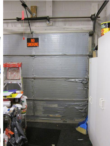
Deteriorating weather-stripping
