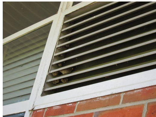
Ground vegetation growing within the exterior walls indicates moisture in the wall and can contribute deteriorating bricks (L). Nesting in non-functional louvers may breed harmful insects (R).
