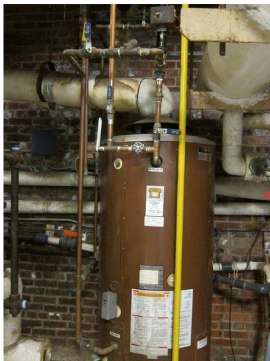
Gas-fired and electric domestic hot water heaters located in the 1938 basement. DHW piping currently lacks insulation.
