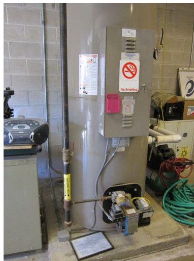
Domestic hot water heater located in the 1999 mechanical room
