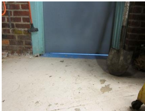
No weather stripping on mechanical room exit (1938 basement exit)
