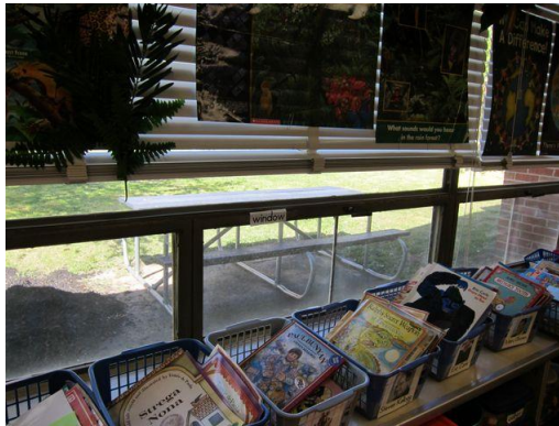
Non-insulated metal frame with single-glazing provides poor insulation to the building(R)
