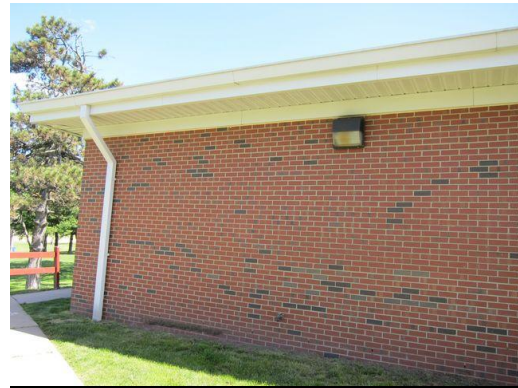
Typical wall pack high pressure sodium fixtures.
