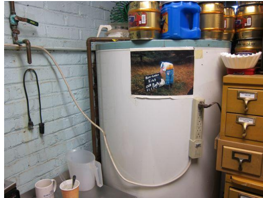
Gas-fired and electric domestic hot water heaters located in the 1938 basement. DHW piping currently lacks insulation.
