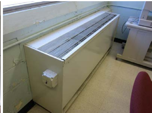
Typical ceiling mounted unit ventilators (L) and typical wall mounted unit ventilators (R)
