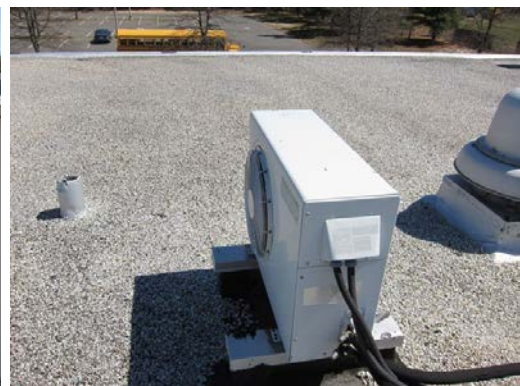
Rooftop unit (L); typical split-DX condensing unit (R)
